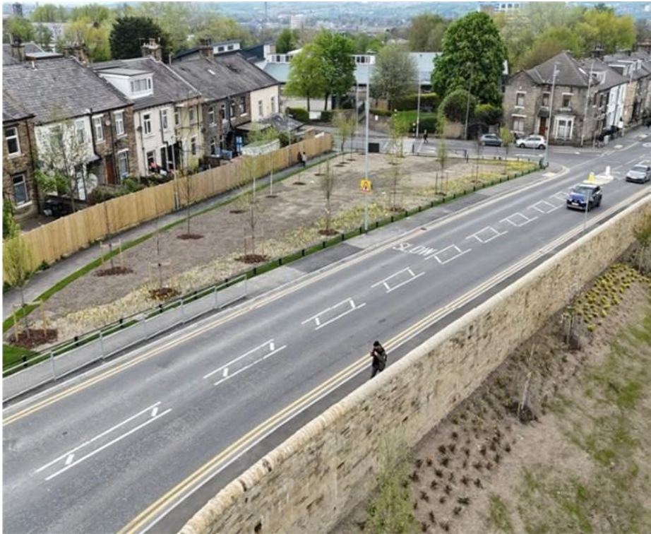
Figure 4.7: SuDs scheme at Great Horton Road (Source: Casey)
