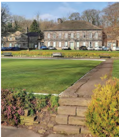
Former Town Hall building, Bingley
