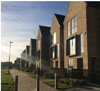
Trumpington Meadows, Cambridge: Small details such as pop-out frames around openings can add interest and depth to an otherwise simple facade.
