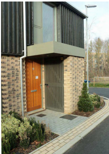
Cornwell Park, Cambridge: Integrated and secure external storage provides space for bins
