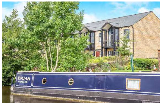
New development designed to respond to its waterfront setting with large windows, balconies and interest in the roof form. Micklethwaite Landings, Bingley.
