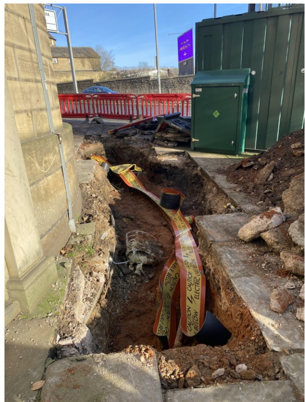
Figure 10: Emergency Repair Works Adjacent to Shipley Airedale Road Air Quality Station
