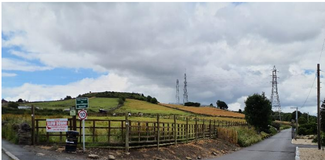
Pylons and mast at Idle Hill.
