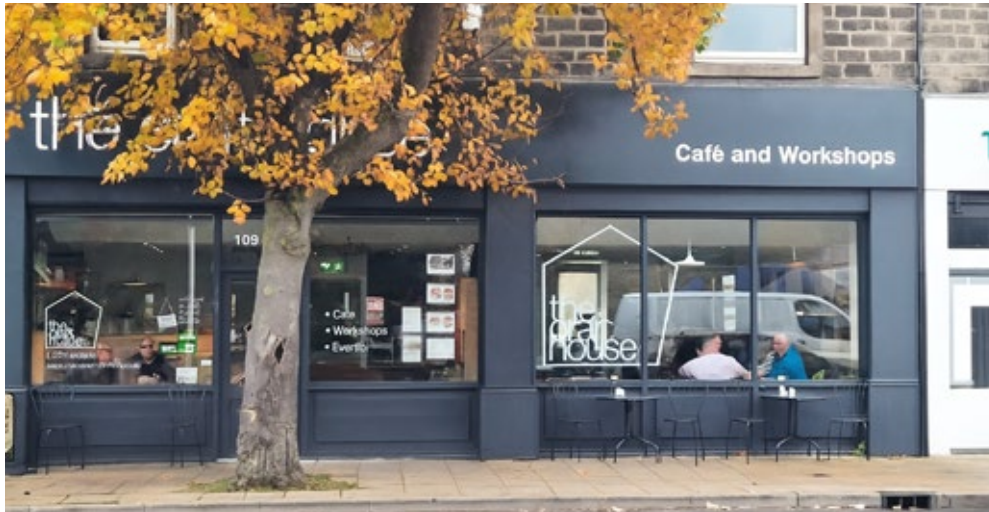
The Craft House, Bingley has a simple but stylish shopfront
