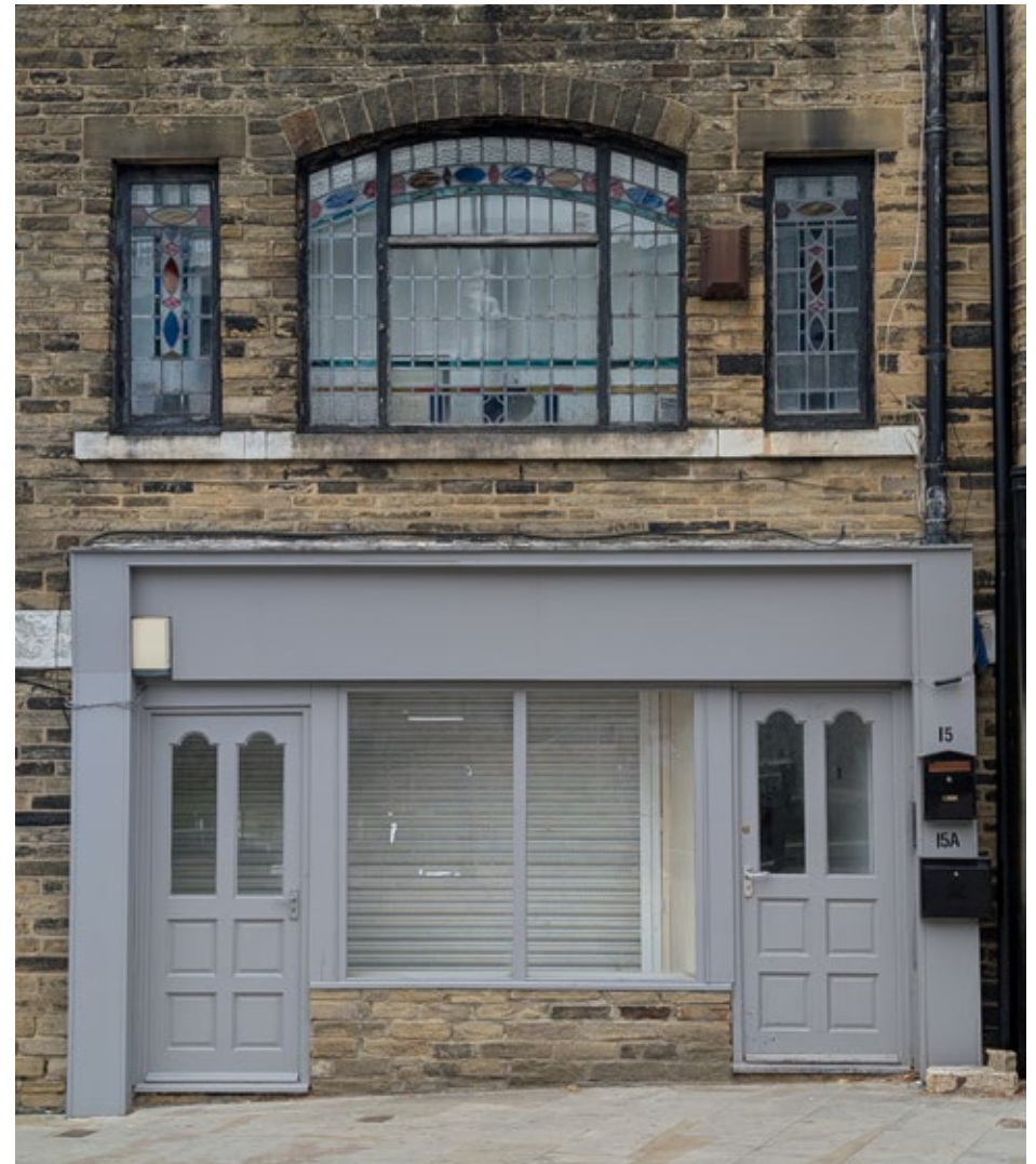
Introducing an additional doorway for upper floor access needs to be carefully considered so that proportions are retained - 15 North Parade, Bradford
