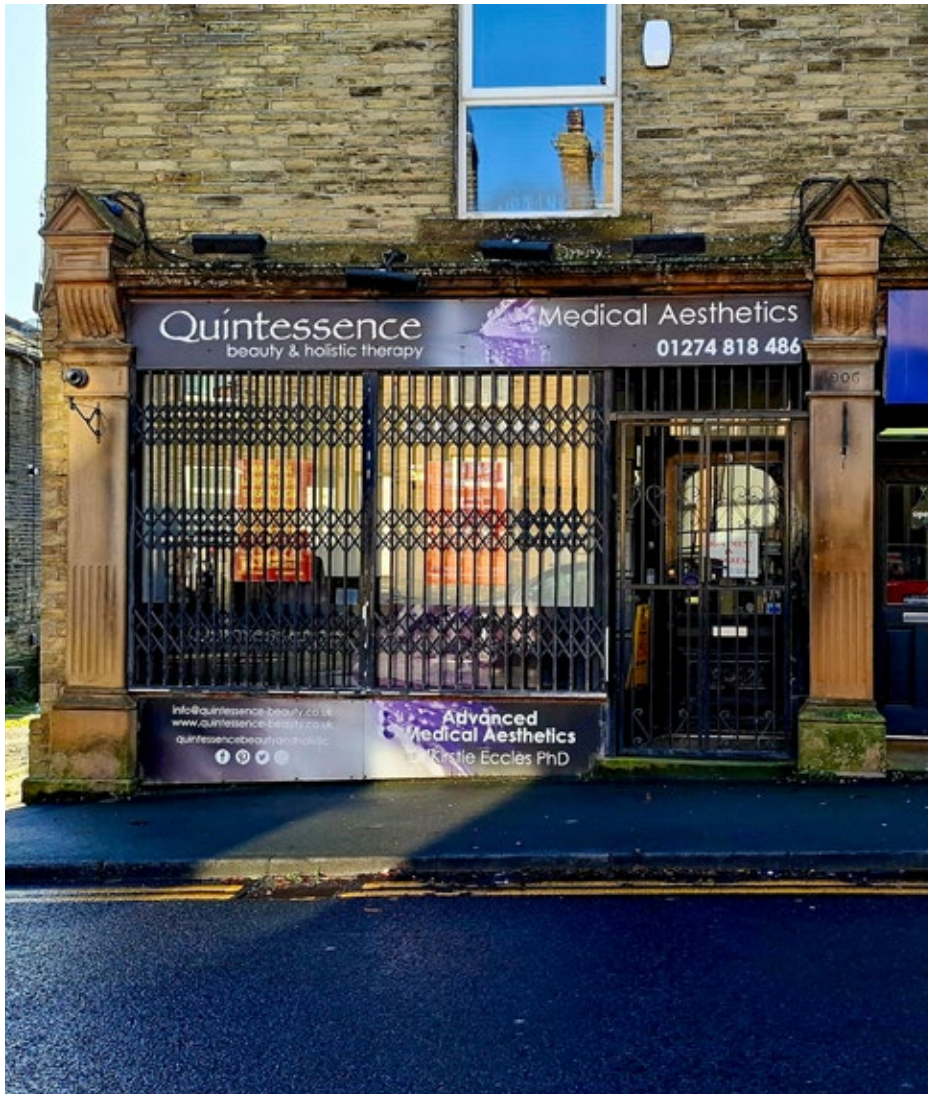
External security grilles on a shopfront in Queensbury
