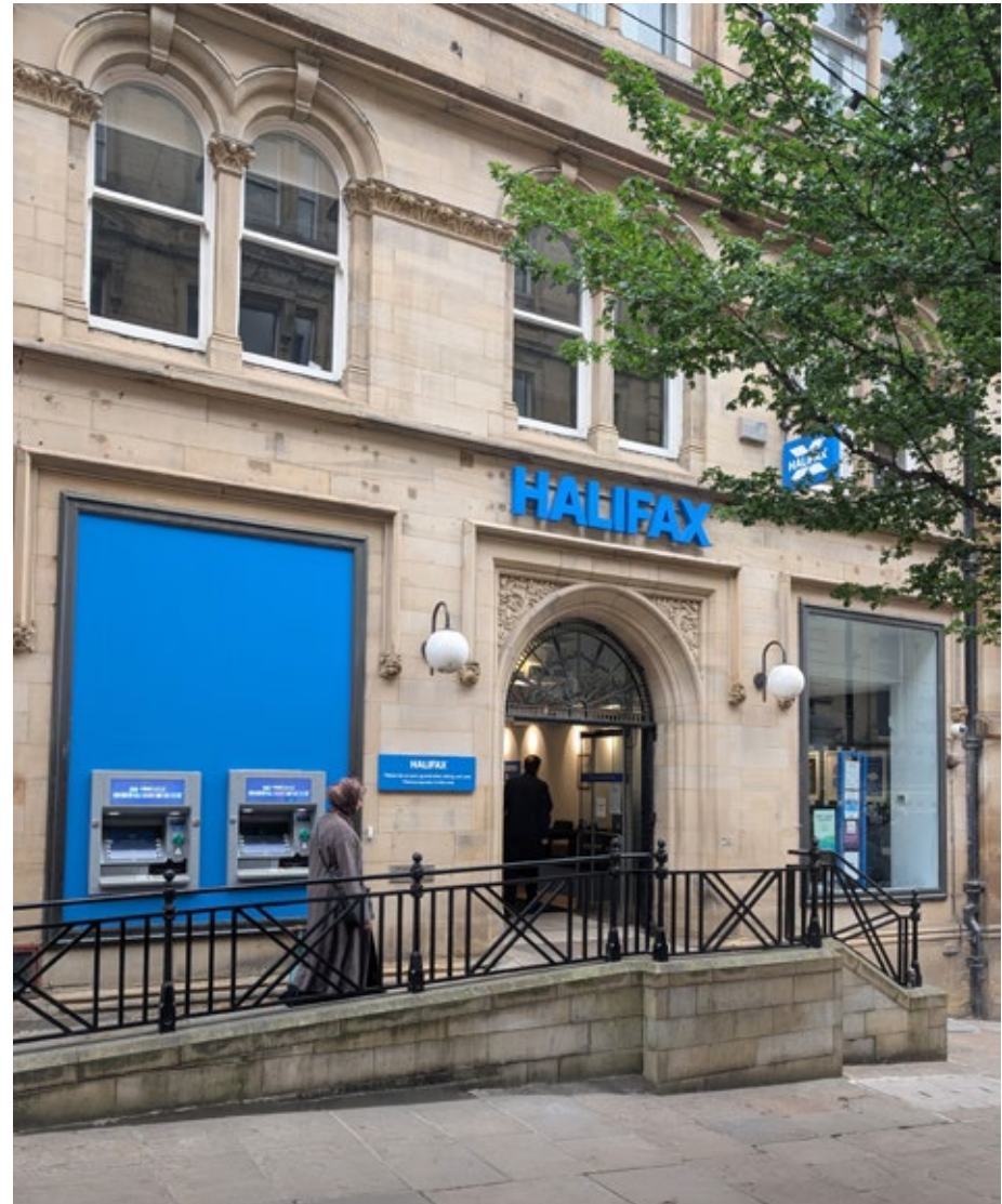
Providing level access on historic buildings can be more challenging but when carefully designed, can work well ( Halifax Bank, Bradford )
