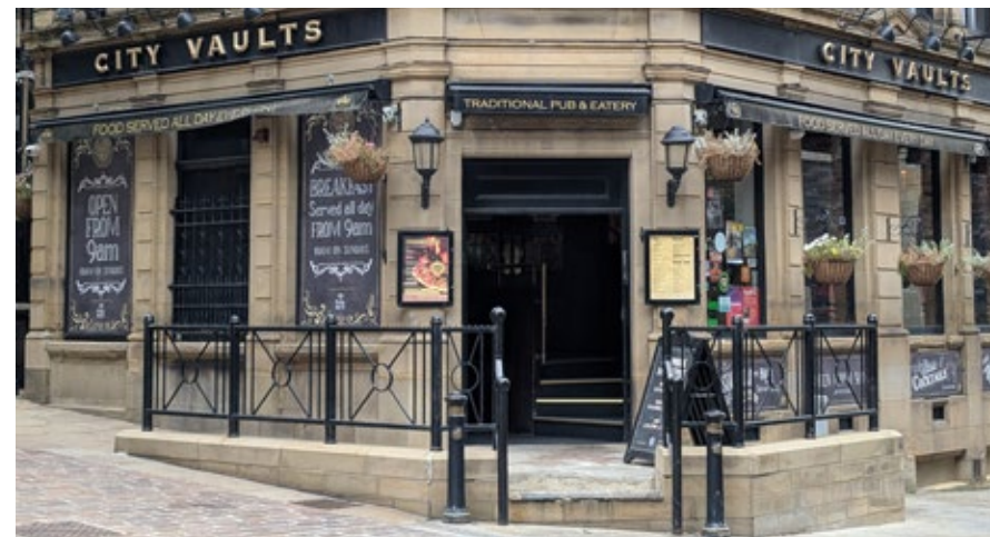
Carefully designed solutions can improve accessibility to existing buildings, such as at City Vaults, Hustlergate, Bradford
