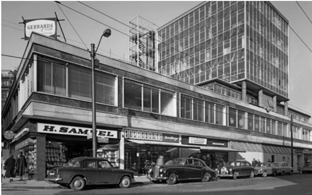
Broadway, Bradford in the early 1960s represented post-war fashions for shopfront design and building styles (Bradford District Museums & Galleries, CBMDC)
