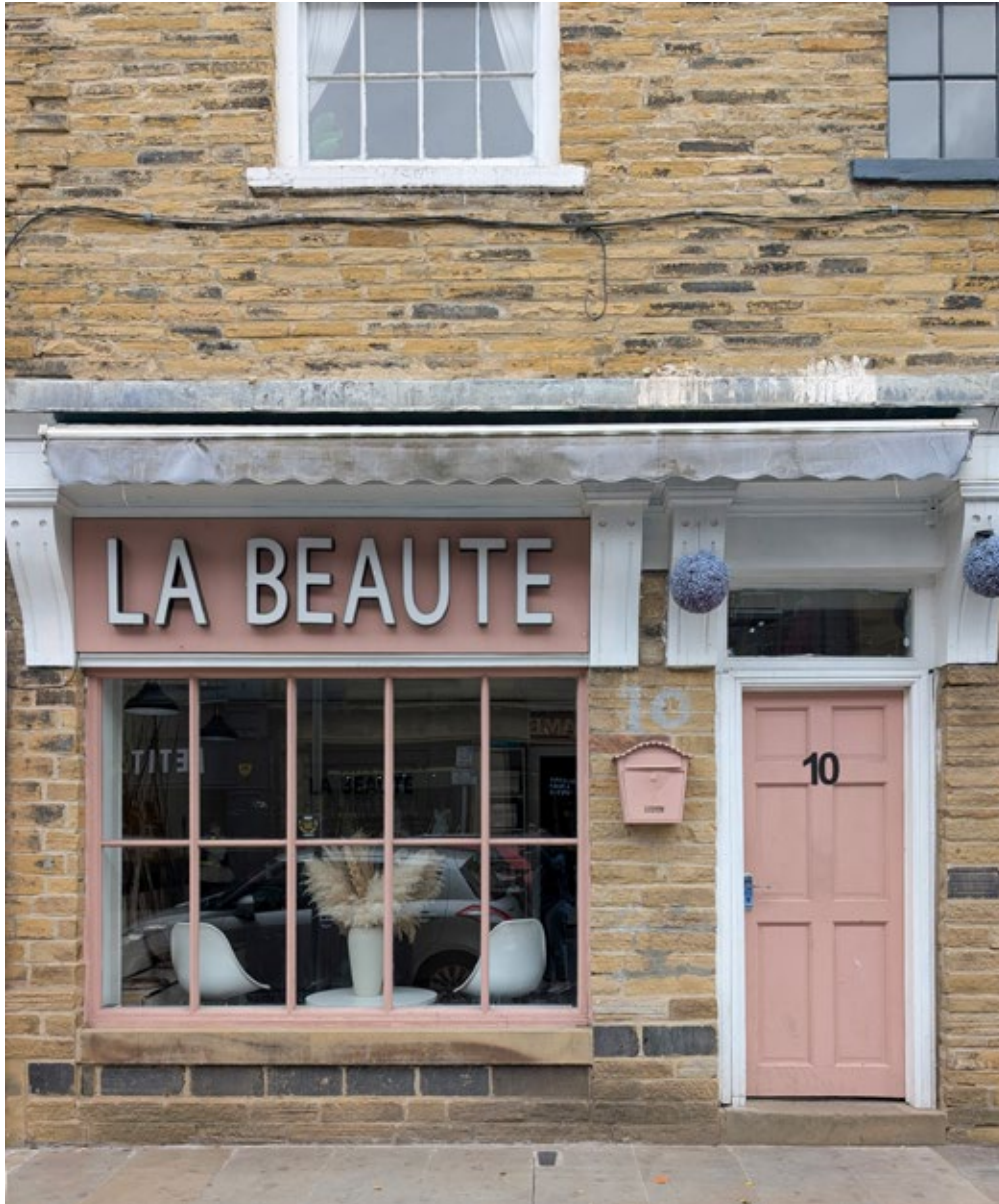
La Beaute, North Parade, Bradford has a simple but well preserved 19th century shopfront. The smaller panes of glass are typical of earlier examples of shopfronts
