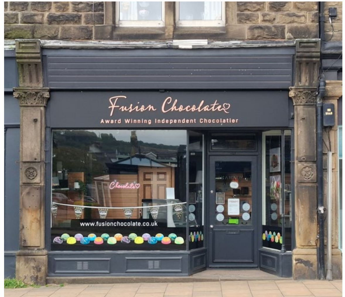
Well integrated ventilation in the stallriser of the shopfront, Fusion Chocolate, Leeds Road, Ilkley
