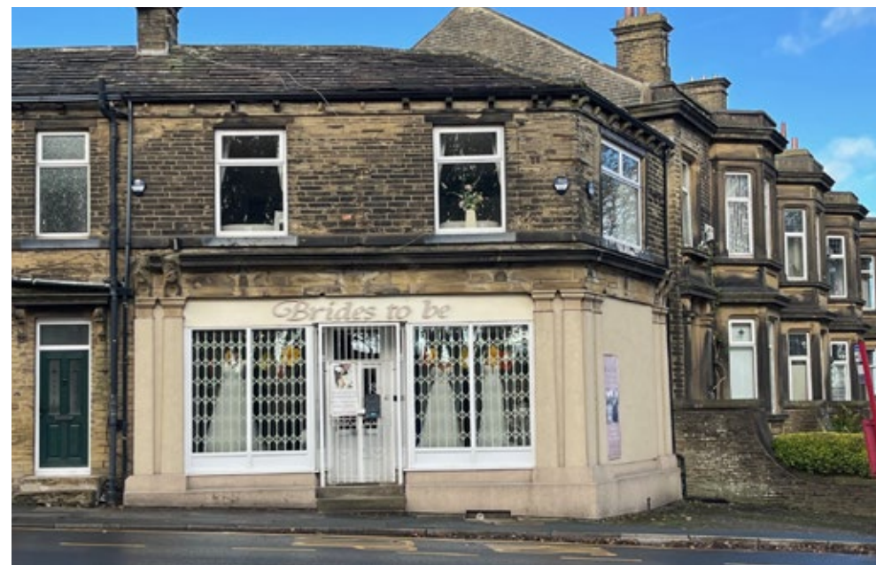
Brides to be, Scarlet Heights, Queensbury – The internal concertina grilles allow for views of the goods when closed and can be neatly tucked away inside the window jambs when open
