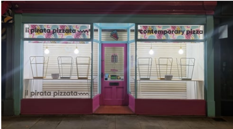
Il Pirata Pizzata, Bingley Road, Saltaire – Example of an internal shutter set back behind the window with simple lighting and display in front contributing to nighttime appeal
