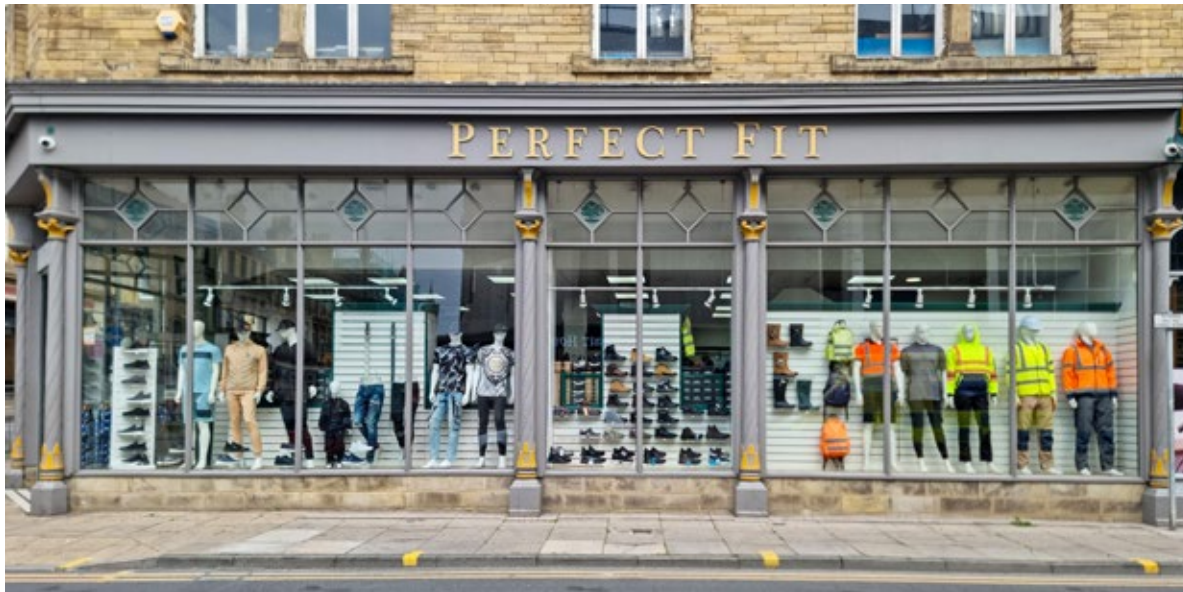
Well detailed example of an Edwardian shopfront at Perfect Fit, Godwin Street, Bradford
