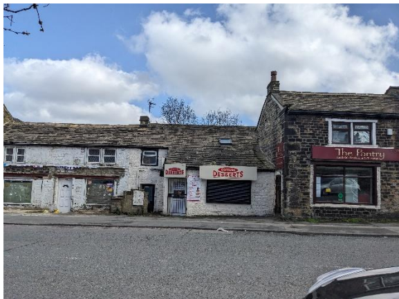
Figure 2: Vacant units along Great Horton Road which detracts from the centre’s attractiveness.
