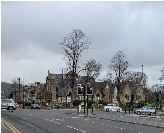
Figure 1: The major £13.7 million Greengates crossroads junction redevelopment, which was completed to reduce traffic congestion and improve pedestrian, cycling, and bus route infrastructure on Harrogate Road and New Line.
