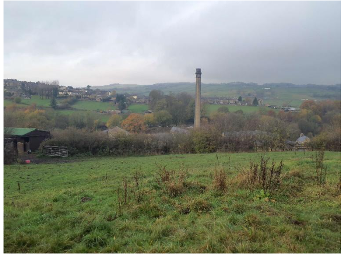
Chimney at Ebor Mill.
