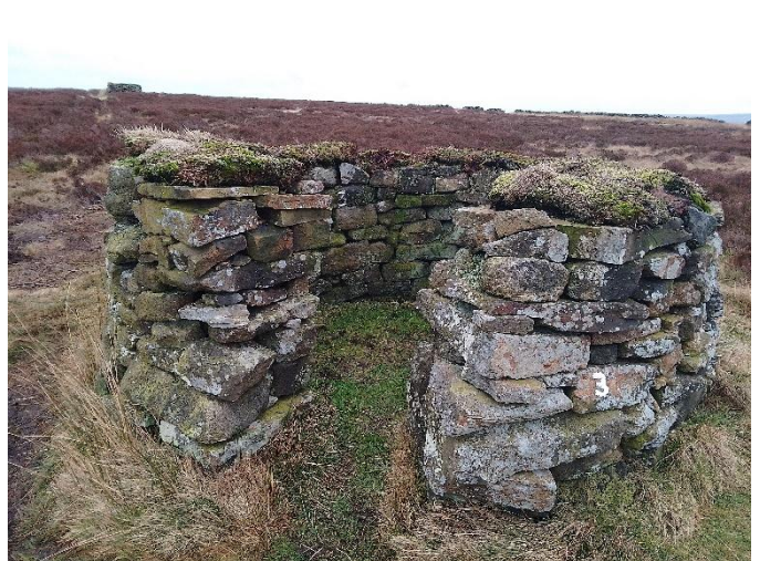
Drystone structures associated with grouse shooting.
