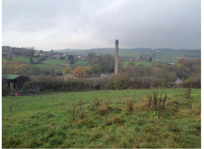
Chimney at Ebor Mill.
