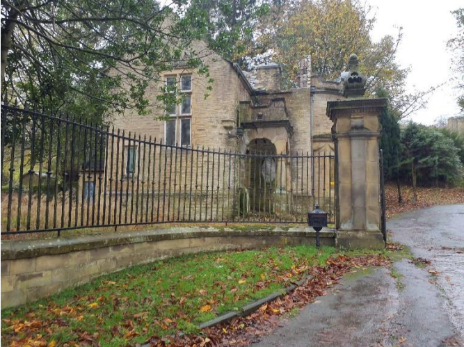
Grade II Gate Lodge Listed Building at Whinburn Registered Park and Garden.
