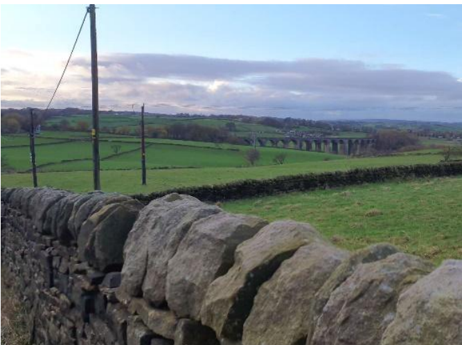
Views towards Hewenden Viaduct.
