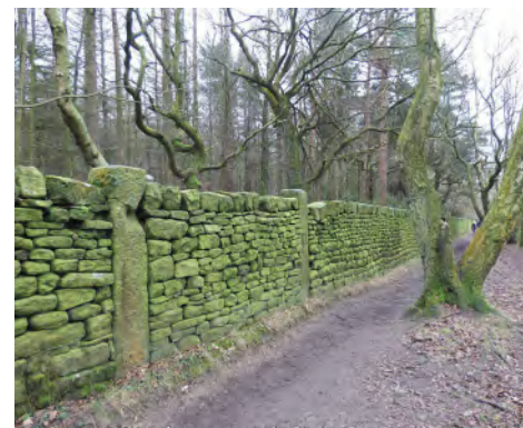
Footpath, St Ive's Estate
