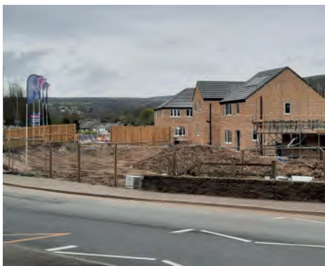
Five Rise Quarter housing development under construction
