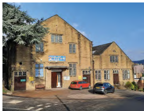
Swimming pool building, Bingley
