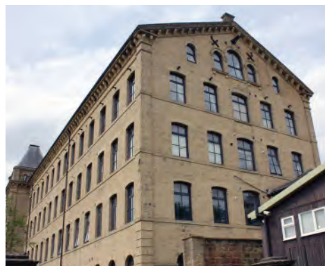
The Locks apartments, Bingley
