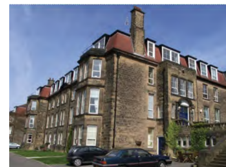
Former college buildings, Bingley
