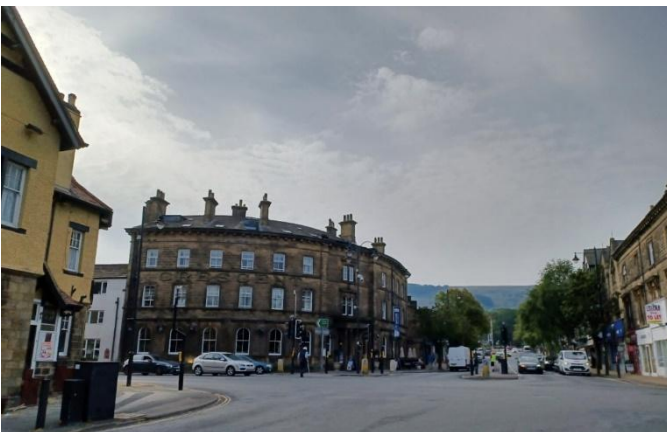
Historic architecture of Ilkley, with the rising form of Rombalds Moor seen in the background.
