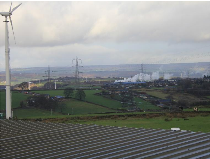
Pylons and wind turbines are prominent features within the LCA.
