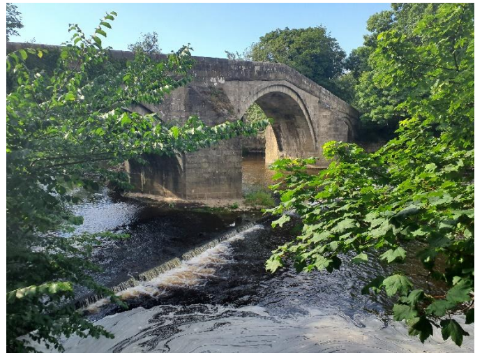
Historic bridge across the River Wharfe within Ilkley Conservation Area.
