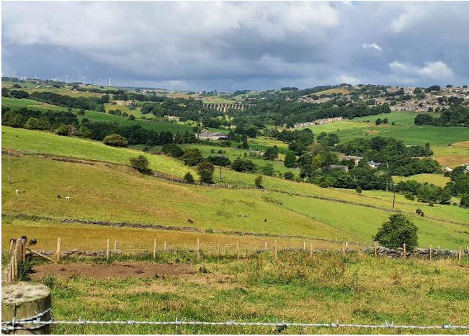
Folds of the valley with the Thornton viaduct widely visible.
