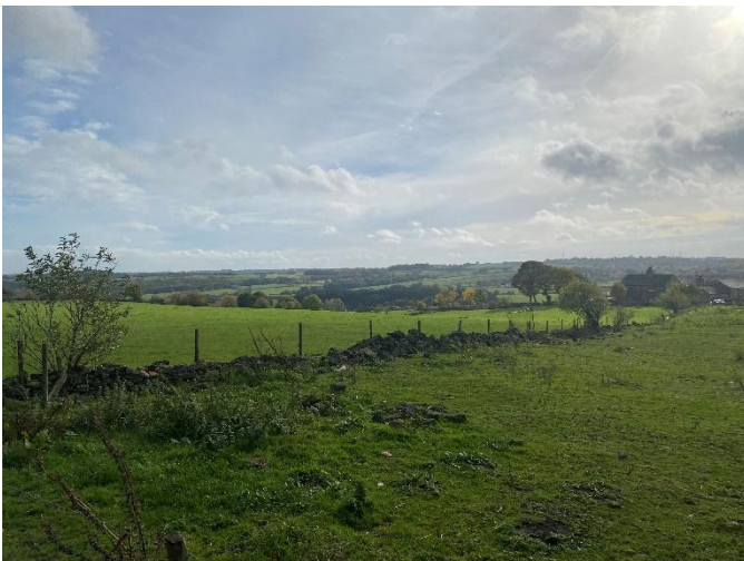
Drystone walls in poor condition and scattered agricultural buildings.
