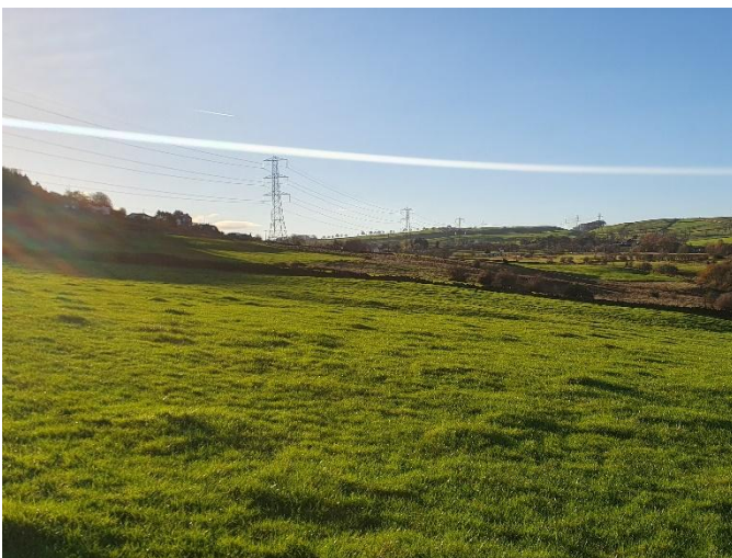
Overhead electricity lines can be seen on horizon.
