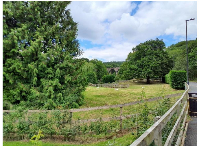
Viaduct at Esholt remnant from rail industry.
