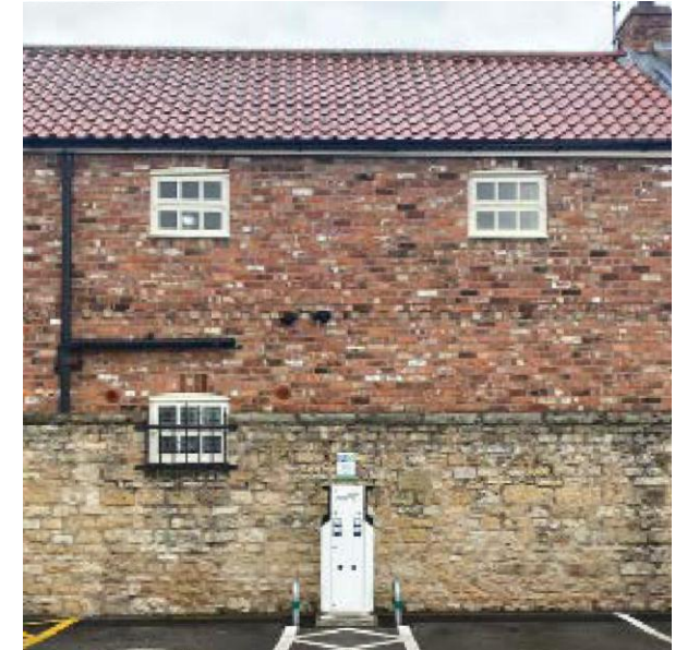
Figure 55: Home electric vehicle charging point located at the side of the dwelling to minimise the visual impact.
