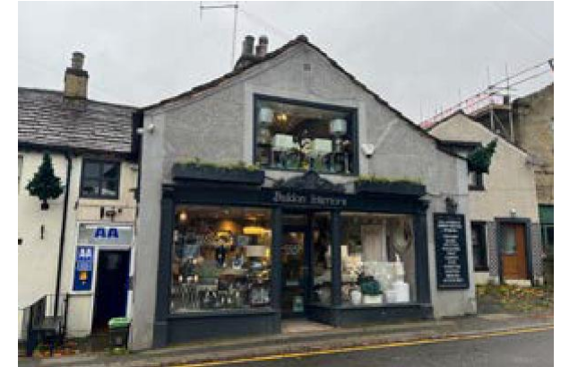
Figure 10: Shop front at Baildon Village
