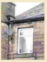
✓ Keep the length of external wiring required to a minimum and if possible, run it closely alongside existing pipes or flues.
