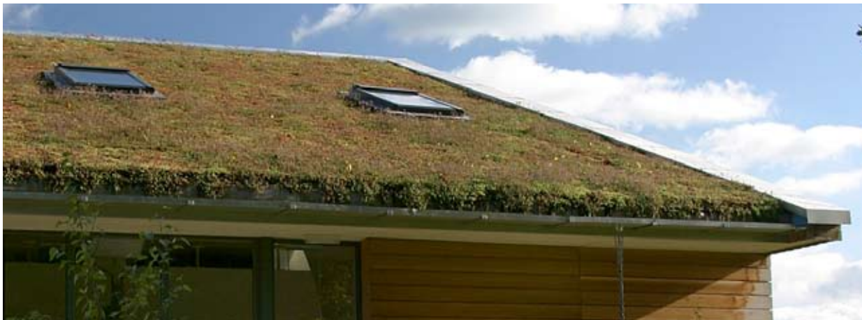
Green roofs are not only attractive and eco-friendly, they can be made to measure and used on most roofs with a slope of 30° or less
