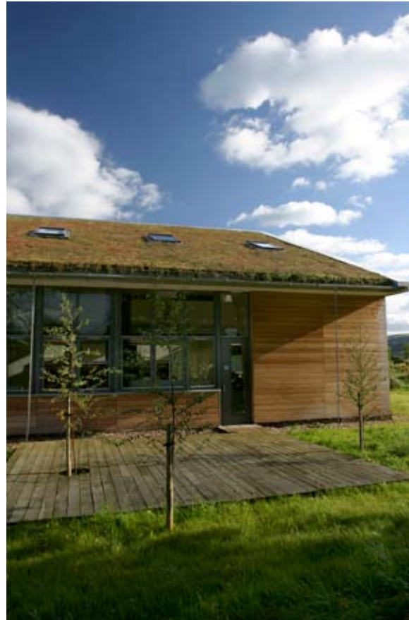
Much of the site of the Ecology Building Society takes the form of a native meadow and wildflower habitat. The sedum roof of the building absorbs rainwater and supplements the internal insulation.
