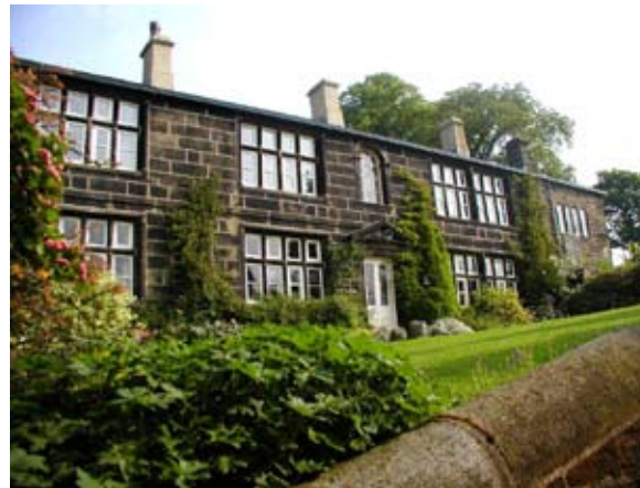
Maximising passive solar heating is not a new concept! Historic buildings, such as this 18th century vernacular house were often built with large windows in their south facing elevations to allow natural daylight and warmth into the building.
