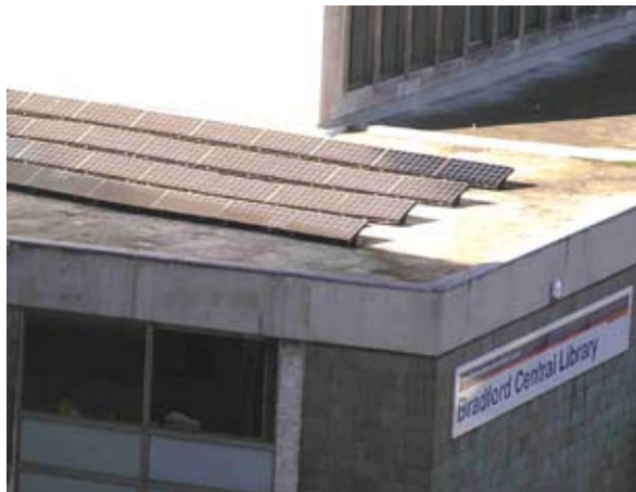
Photovoltaic panels make good use of the flat roof at Bradford Central Library.
