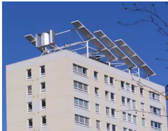
This recently refurbished block of flats in Bradford city centre has been fitted with a silent wind turbine (on the left) which helps power the building.
