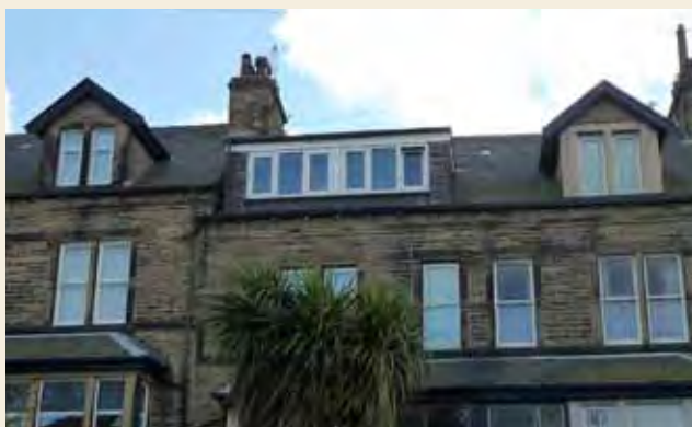
Figure 37: Unacceptable - original dormers should not be replaced by box type dormer windows
