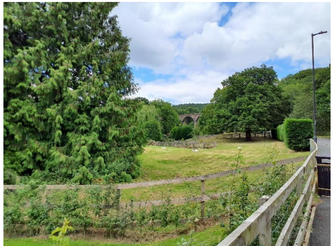
Viaduct at Esholt remnant from rail industry.
