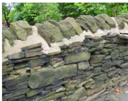
Far right: Poor use of signage. Right: Poor pointing that damages the wall.
