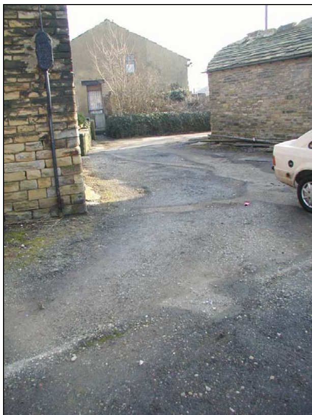
The conservation area contains no street surfaces made of natural stone. The tarmac surface of the pathway behind Snowden Road is in a poor condition as well as inappropriate in terms of material.
