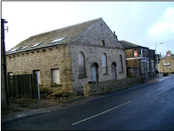
Former Methodist Chapel, Main Street (unlisted).
