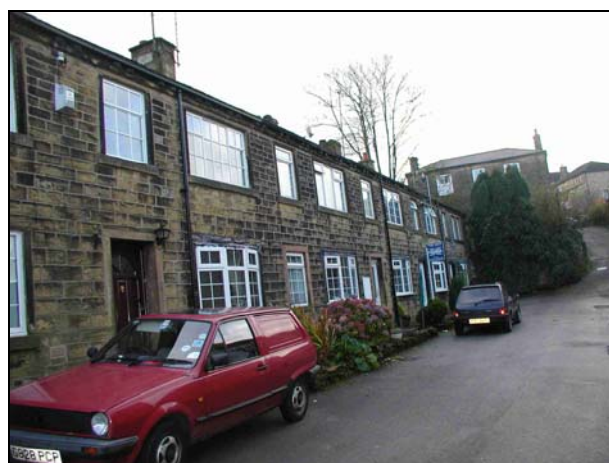
Cranford Place (unlisted) was built to house workers at Albion Mill in the 1820s. Much of the integrity of this row has been lost through the removal of its original window detailing. The former mill master's house, Providence Hall (unlisted) is uphill in the background.
