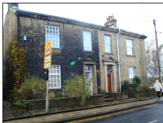
The cleaning of stone can break the sense of unity, particularly when the property forms part of a group such as this pair of houses at 134-136 Main Street.
