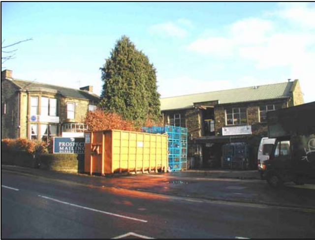
Well House and Well House Mill accommodate a range of commercial uses and bring life and activity to the conservation area.
