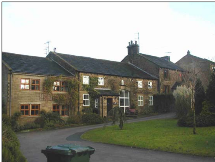
Greenwood House and Turvy Barn (unlisted) is another farm complex in the conservation area dating from the eighteenth century. The conversion to a residential use has occasioned several changes including the glazing of the barn archway and the addition of a stone porch. The element to the left is new build.
