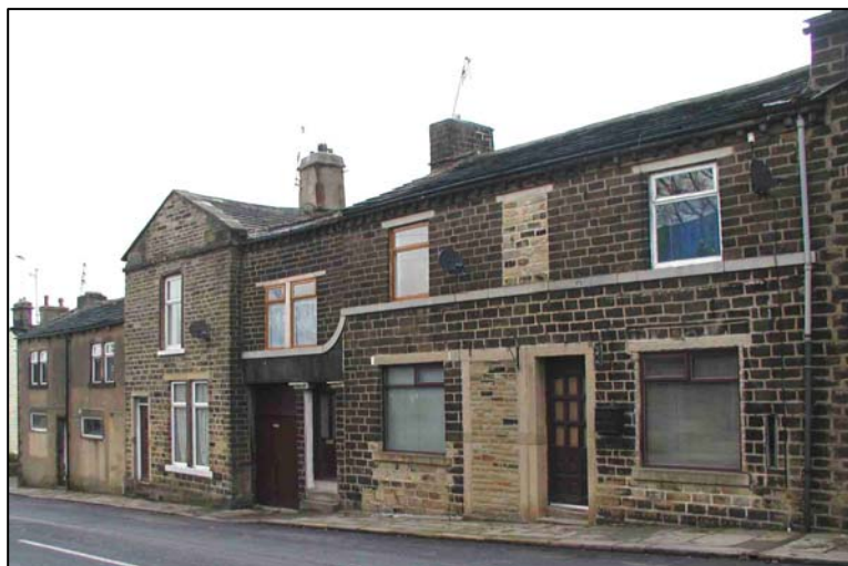
57-67 Main Street (unlisted) lack consistency due to the insertion of different types of windows, and renders and the removal of mullions and other changes to the fenestration.
