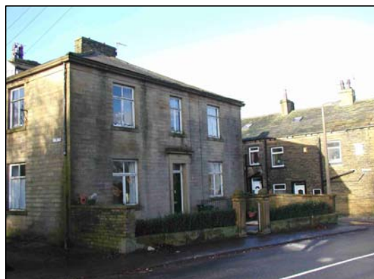
222 Main Street (unlisted) features Regency-style detailing.
