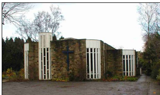
St Matthew's Church (unlisted) is an innovatively designed building from 1972 which makes good use of natural materials.
