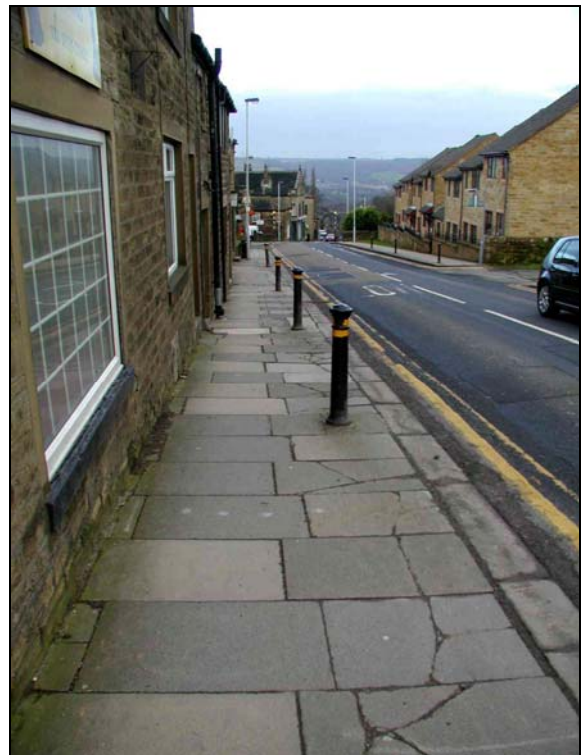
The use of concrete for street surfacing and the use of off-the-peg street furniture such as these bollards provide a poor contrast to the local stone and the thoughtful design of the buildings.
