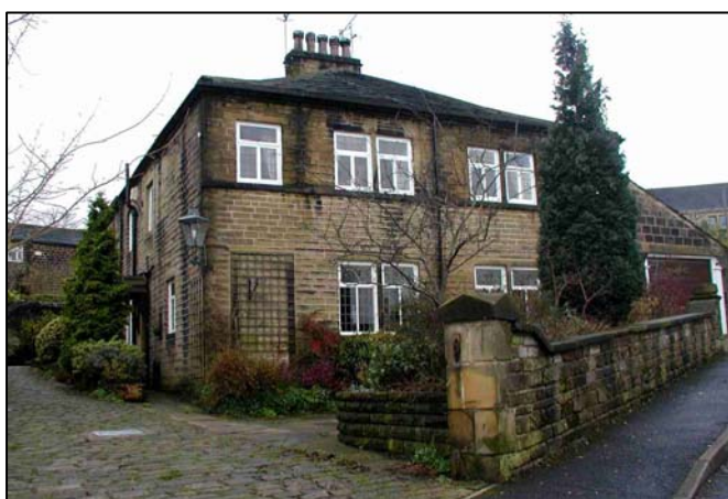
Spring Farm (unlisted). This hipped gable end is a nineteenth century extension. The rest of the laithe dates from the eighteenth century. The timber casement windows with lead and stained glass date from the early twentieth century.
