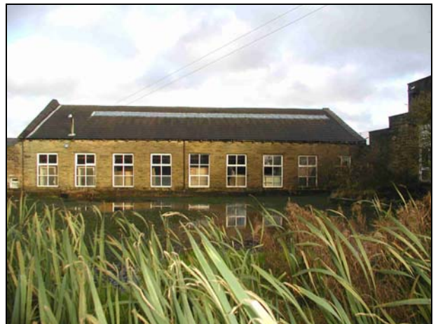
Ling Bob mill pond is one of several water features in Wilsden Conservation Area.
