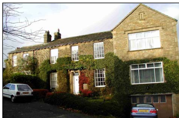
The original building to North House (unlisted) on Wilsden Hill Road (in the centre of this photo) is strongly Georgian, with eight-pane sash windows arranged in a symmetrical grid pattern.
