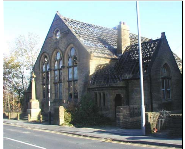
The former Wesleyan Sunday School (Grade II listed) now has a certain future as it has found a new use.
