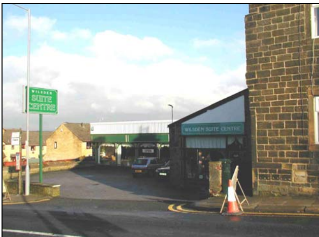
Wilsden Suite Centre occupies what was formerly part of Albion Mills. While reinforcing Wilsden as a retail centre, its design, layout and use of materials undermine the conservation area.
