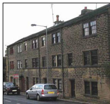
71-77 Main Street (Grade II listed) are part of an L-shaped fold of three-storey cottages. The archway below number 73 leads to 1-5 Garden View.
