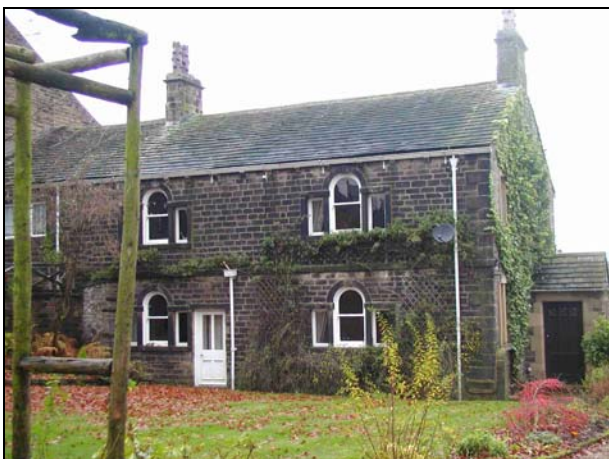
Spring Mill House (Grade II listed) is a former farmhouse which was refronted in 1780, by which time its owner had prospered through the manufacture of textiles. The Venetian windows are an unusual classical feature on what is otherwise a vernacular building.
