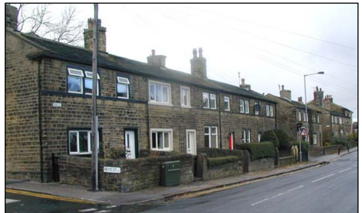
These cottages at 138-154 Main Street (unlisted) date from the early nineteenth century. Their flat, uniform frontage gives them a strong sense of unity.
