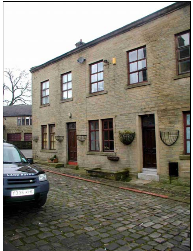
Wilsden Mechanics Institute (Grade II listed) has been successfully converted to six dwellings with minimal changes to the building's exterior, though the new windows lack the detailing of the originals.
