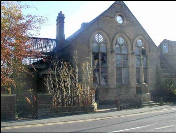
The former Wesleyan Sunday School (Grade II listed) stands vacant and roofless.
