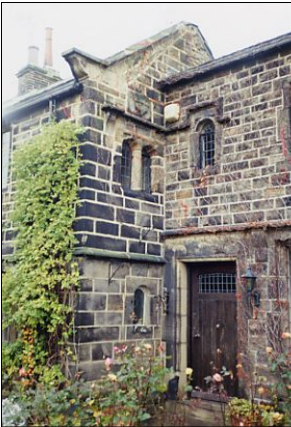
The vernacular detailing of kneelers, chamfered openings, hoods and dripmoulds are found at The Manor House and on many other buildings in Tong.
