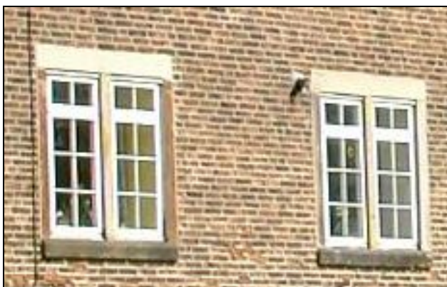
Left: Tong Hall is one of the earliest examples of the use of sash timber sash windows in the country. This type of window opening was prevalent in England for the 200 years or so after its introduction. Below: Here synthetic windows with a non-traditional opening have replaced the timber sash windows. These windows are also set quite close to the wall. The original sashes would have been more recessed than these replacements.
