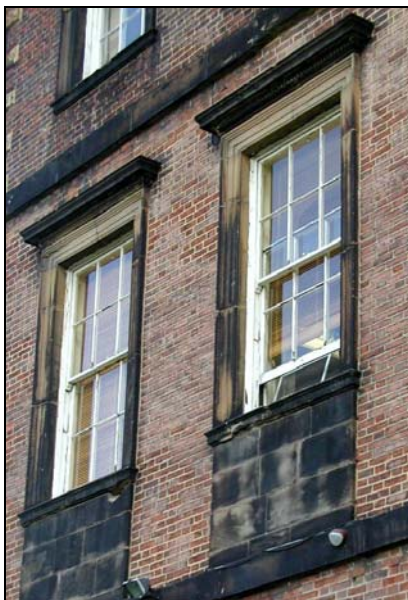
Left: Tong Hall is one of the earliest examples of the use of sash timber sash windows in the country. This type of window opening was prevalent in England for the 200 years or so after its introduction. Below: Here synthetic windows with a non-traditional opening have replaced the timber sash windows. These windows are also set quite close to the wall. The original sashes would have been more recessed than these replacements.
