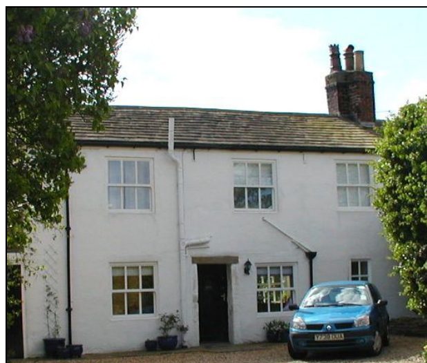
24 Tong Lane (unlisted) is at the end of a row of estate workers' cottages built in the 18 th century. Underneath the render are the same red bricks visible on the chimney. The retention of the stone roof and three-pane Regency-era sash windows gives this cottage a historic appearance.
