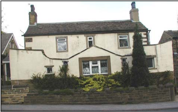
13 Tong Lane (unlisted) might well be a historic building given that it has 17 th century quoins at its west end and 18 th century quoins to the east. However, the rendering of the walls and the removal of original features such as the windows makes this impossible to discern.
