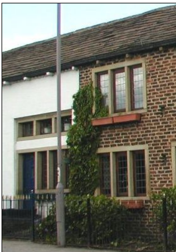
It is a shame that many of the handmade Georgian-era brickwork in Tong has been covered with renders which drastically alter the appearance of the building and undermine the unity of groups of buildings such as this row of cottages.
