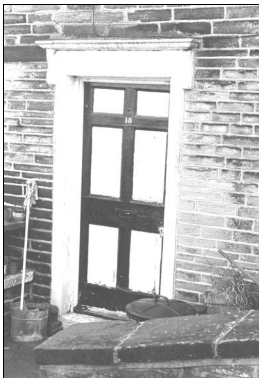
Traditional doorway with a cornice carried on console brackets.
