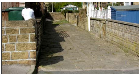
Stone setts to the rear of Croft Street. Very little traditional highway surfacing remains in Steeton, standard modern materials such as tarmacadam have replaced most.
