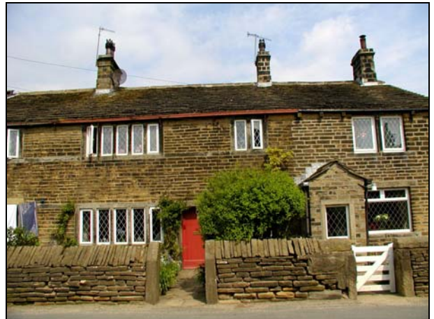
Nos. 78-82 Main Street, like most buildings in the village, are roofed in local stone slate. This traditional material, now becoming rare, is an important characteristic of Stanbury.
