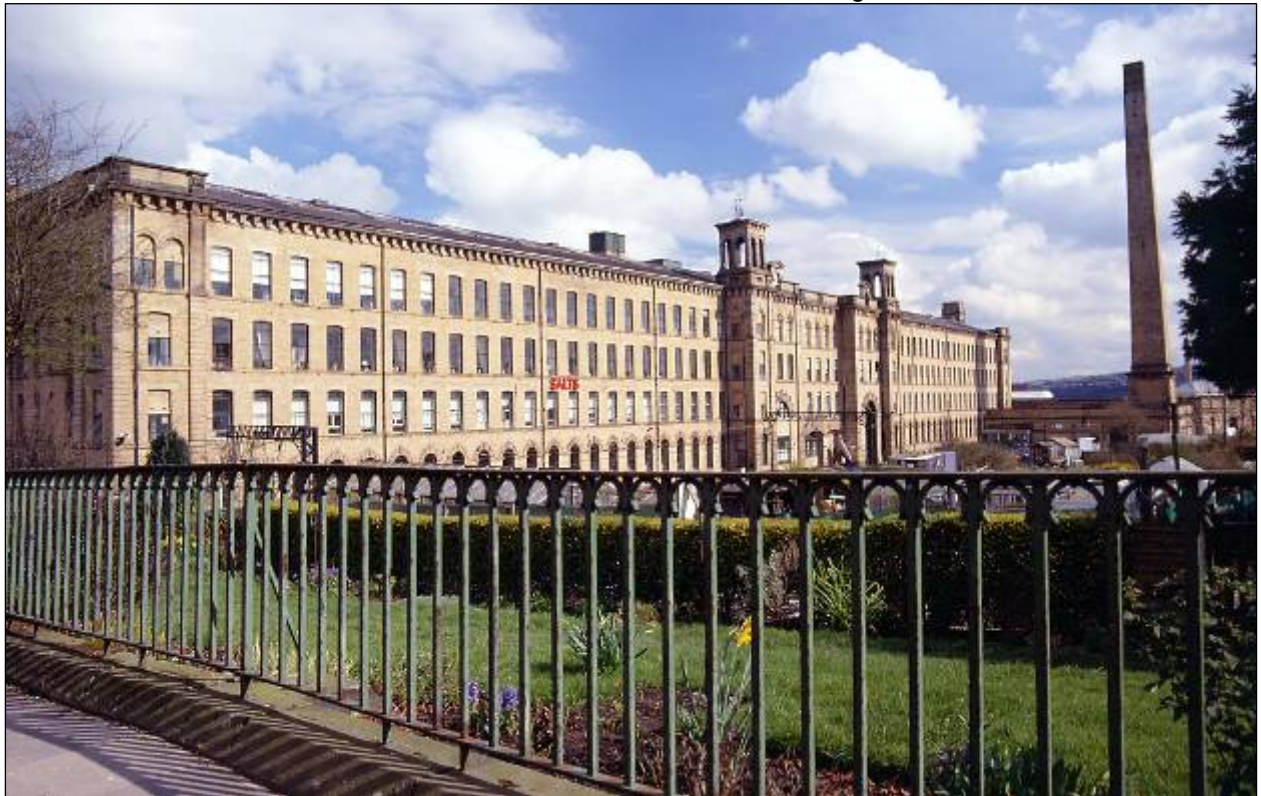
Salts Mill – built as an integrated mill to carry out all of the processes of textile production under one roof. It was innovative in design and incorporated fire-proofing and health and safety measures. This is one of the most important buildings of the village and its raison d'être. The level of architectural treatment of the building is exceptional and would have been a fine advertisement for the company and continues to be a focal point of the village.
