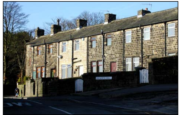
The terrace of 19 th century houses to the north of Oakworth Hall have good stone slate roofs but sadly have lost many of their original features.
