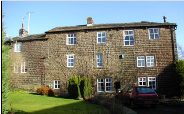
47-51 Oakworth Hall were formerly known as Haggas Fold. Now in residential use, the upper floors were formerly used for textile manufacture.
