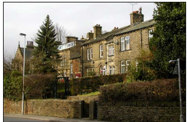
The large houses on the north side of Lidget were built for affluent Victorian families around the end of the 19 th century.
