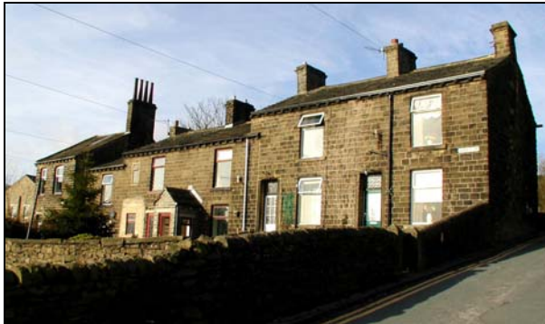
Oakworth Terrace, a group of late 19 th century cottages, has an interesting and varied roofscape.
