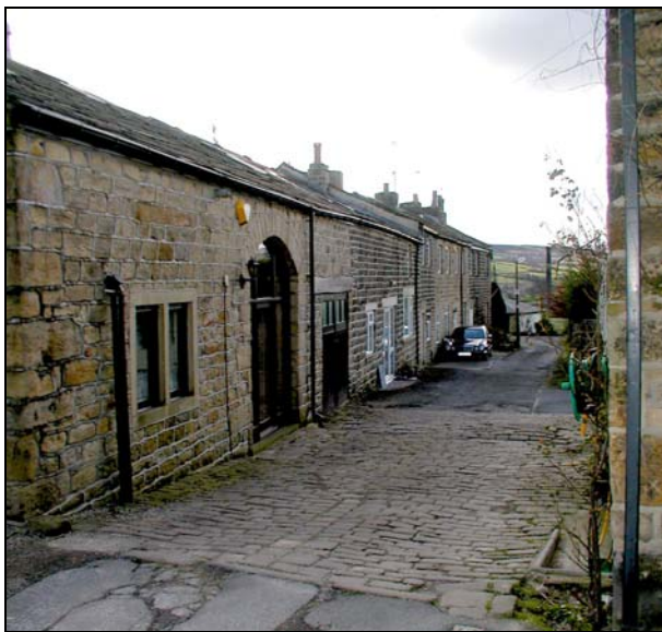
The north elevations of the cottages and converted barns at Dockroyd display much traditional character.
