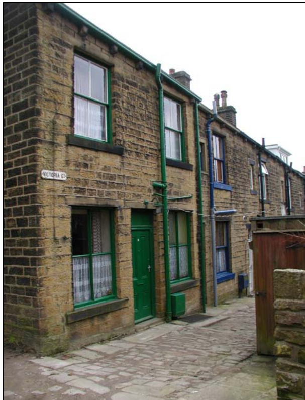
The rear elevations of the houses on the north side of Victoria Road display much traditional character and have retained a higher degree of original features than the front elevations.
