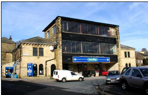
The building used by the Co-operative Society once formed the stables and coach house to Oakworth House.
