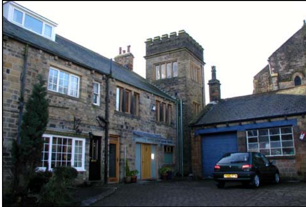
The north elevations of the Manor Tower and Coach House; the tall square tower is an interesting feature of the group.
