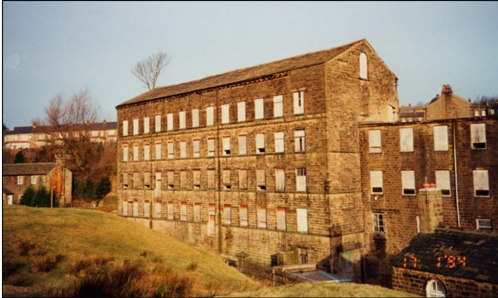
Oakworth Mill, a Grade II listed building, is sadly no longer standing. It was demolished after a fire in early 2000.
