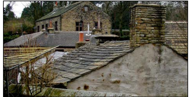
Stone slate roofs are the traditional form of roofing material on most buildings constructed before the middle of the 19 th century.
