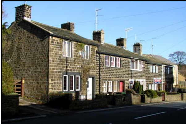
14-22 Goodley is a group of interesting early 19 th century cottages that were probably built for the textile workers.
