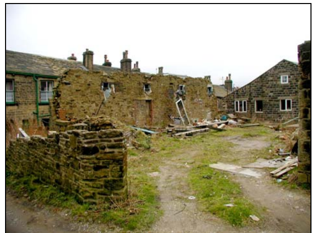
The former site of Lidget Mills is a potential hazard and the site urgently requires a new use.
