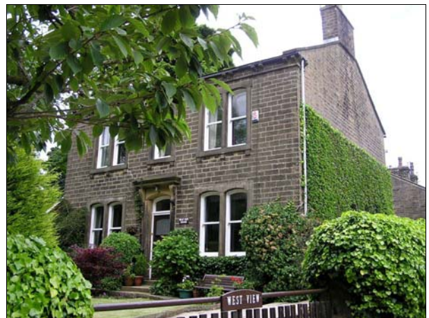
West View, Station Road retains key features and details. This Victorian villa is a key unlisted building in Oakworth Conservation Area.
