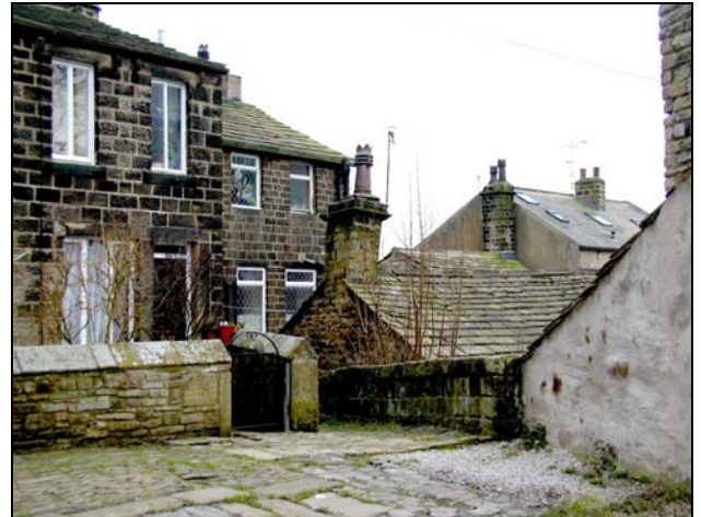
From Hall Street there are good views and vistas across the roofscape of the houses on Clough Gate.
