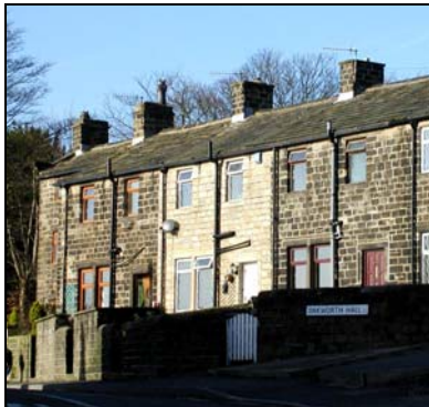
Stone cleaning individual buildings in a row or terrace can create a patchwork effect that harms the unity of the group.
