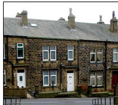
Blue slate roofs are commonly seen on many of the late 19 th century terraces in Oakworth. It has a darker, smoother profile than stone slates.
