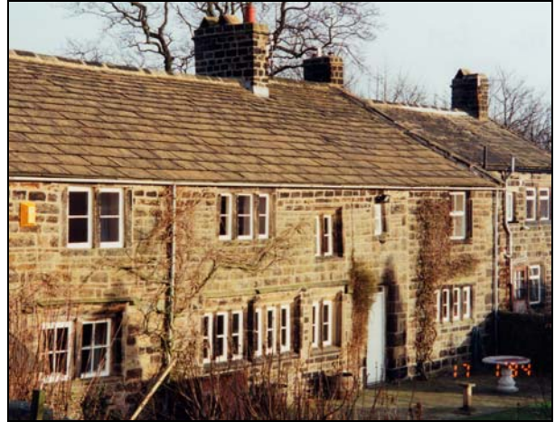
Clough House Farm, a Grade II listed building was probably built around the end of the 17 th century.
