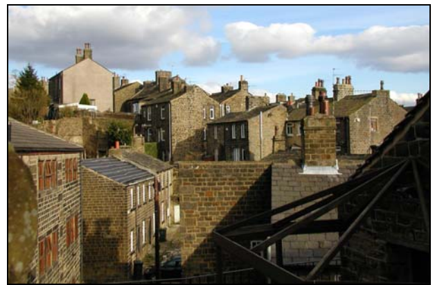
The sloping topography of the conservation area allows good views across the roofs of the houses around Clough Lane.
