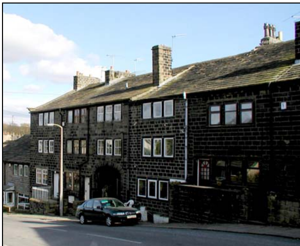
The cottages at the southern end of Bridge Street, 39 to 43 are a storey taller than the cottages further down the hill and consequently make an important contribution to the townscape.
