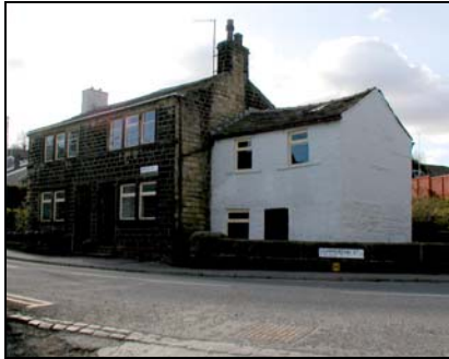
2 and 4 Bridge Street are located opposite the junction with Mill Lane. Their varying heights and stone walled garden adds interest to the streetscape.
