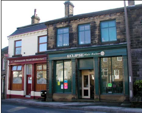
The traditional shop fronts on the properties adjacent to Oakworth Hall make a substantial contribution to the historic interest and character of the group.
