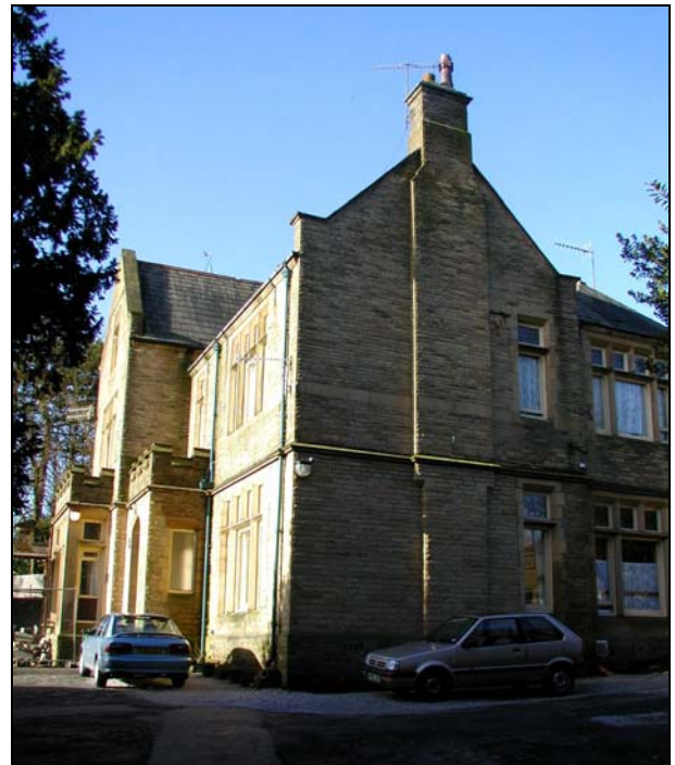
Oakworth Manor was built around the start of the 20 th century and is a key unlisted building in the conservation area.
