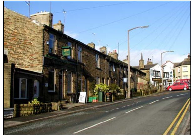
The cottages on the west side of Commercial Street probably date back to the early 19 th century and are of considerable townscape value.
