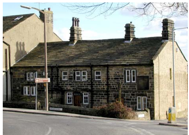
The north elevation of Oakworth Hall is set slightly below the level of the road and displays a number of interesting vernacular features.
