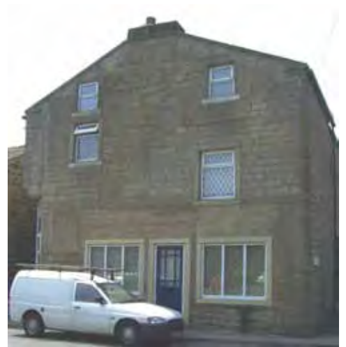
Inappropriate pointing and windows
