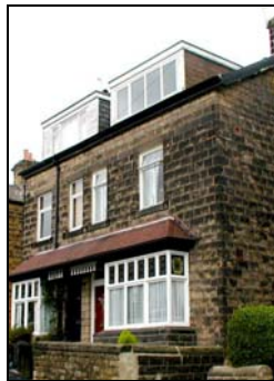
The flat-roofed dormer windows on the front roof slope of these semi-detached dwellings is an unsympathetic alteration, a smaller pitched roof window would be less intrusive.
