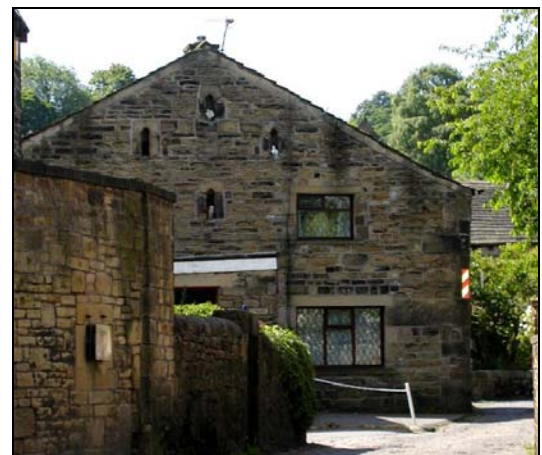
Gable end of Keelham Barn (no. 14) retains the small arched openings which acted as ventilators and as a dovecote.
