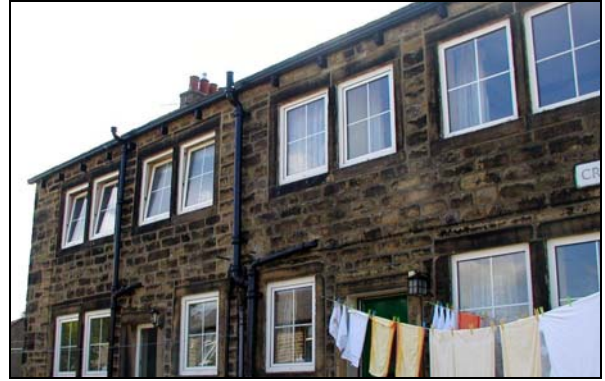
An example of less sympathetic replacement windows in a listed building – the use of unnatural materials and the poor detailing to the frames has an overly dominant impact on the simple character of the house.
