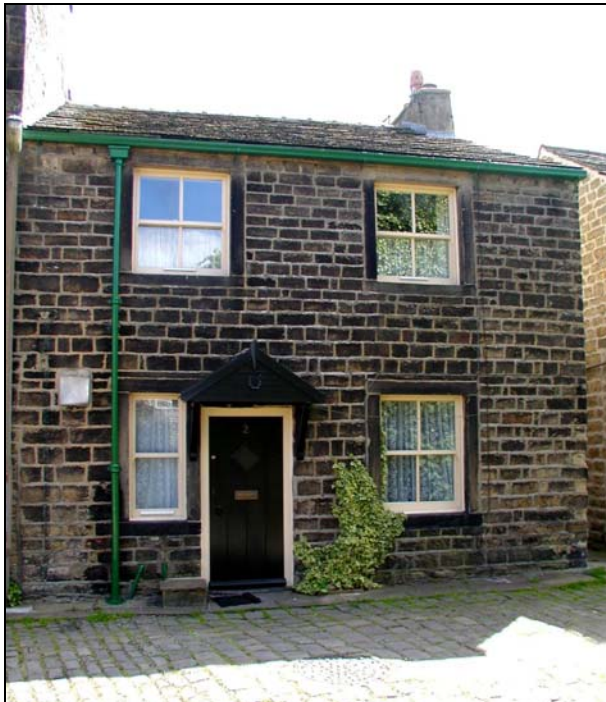
2 Croft House Lane is a good example of a vernacular building which has been carefully maintained. Where original features have been replaced (in this case the windows), it has been done in a sympathetic manner which has not affected the building's character.
