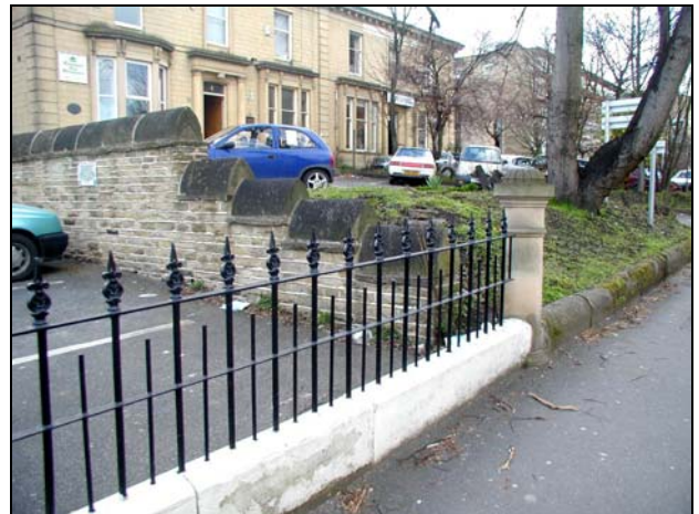
Claremont is mostly lined with low sandstone slabs walls, which, in the example shown has been painted, but good replacement railings have been recently added. Note also the original stone pier and the coped retaining wall.
