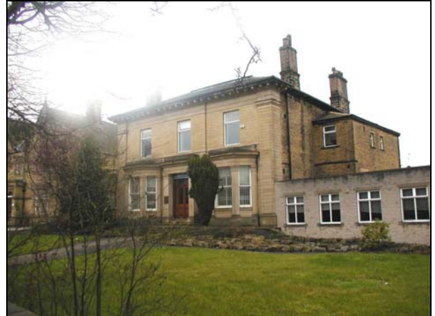
66 Little Horton Lane is one of the few villas to retain any kind of front garden, which helps the buildings to retain its domestic character.
