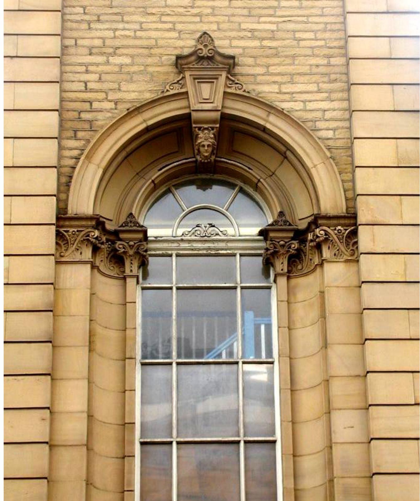
Sandstone 'brick' wall with traditional inconspicuous lime based mortar flanked by smooth faced ashlar stonework with carved ashlar window surrounds at Bradford College Library.
