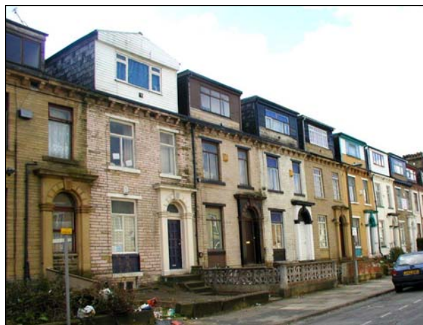
The painting of one or more houses in a terrace such as this one creates a strong visual inconsistency between neighbouring dwellings and conceals the natural stone. Note also the modern dormers which have radically altered the appearance of the houses.
