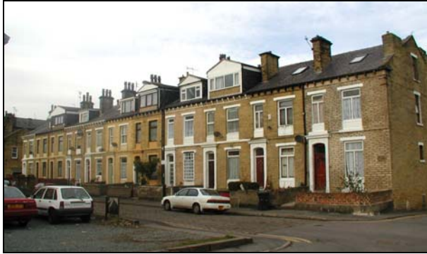
3-23 Ann Place, located on the north side of the road, have been much altered over the years.
