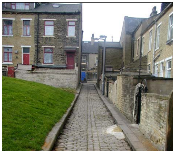
Back Giles Street is a characterful lane that is surfaced with stone setts. At its junction with Little Horton Lane, the road is narrow and lined closely with buildings.
