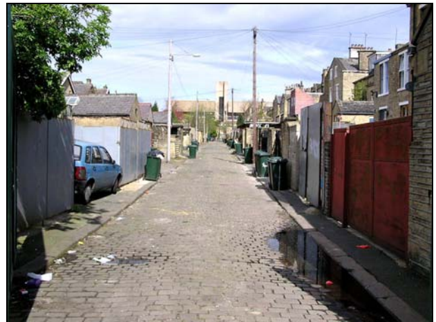
Back Ashgrove (West) is a linear, setted back street which is visually marred by the inconsistent appearance of the structures which line it.
