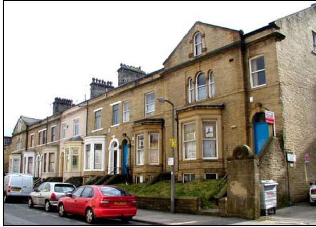
4-16 Grove Terrace (Listed Grade II) is a symmetrical, Italianate row which stands on top of its raised basement storey.
