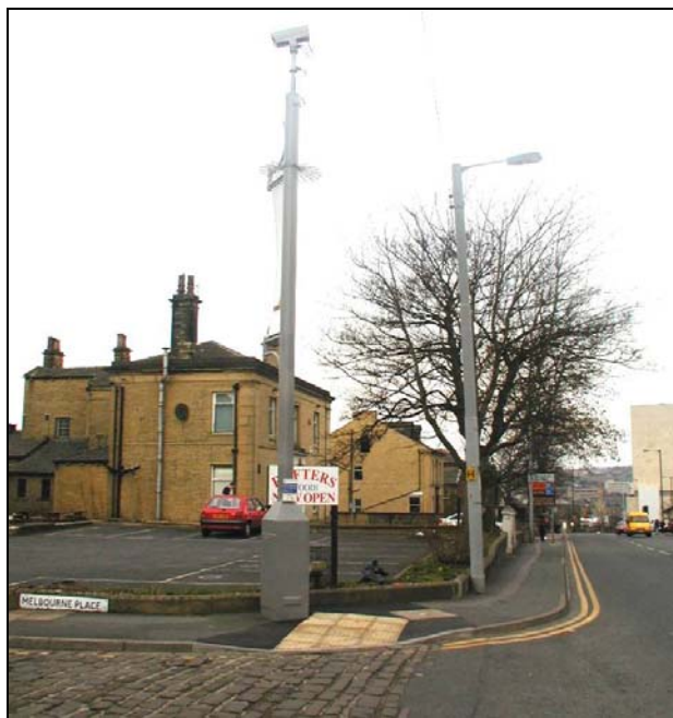
Unsympathetic interventions such as the streetlights, crossing and CCTV installation stand cheek by jowl with traditional stone streetscape and boundaries.
