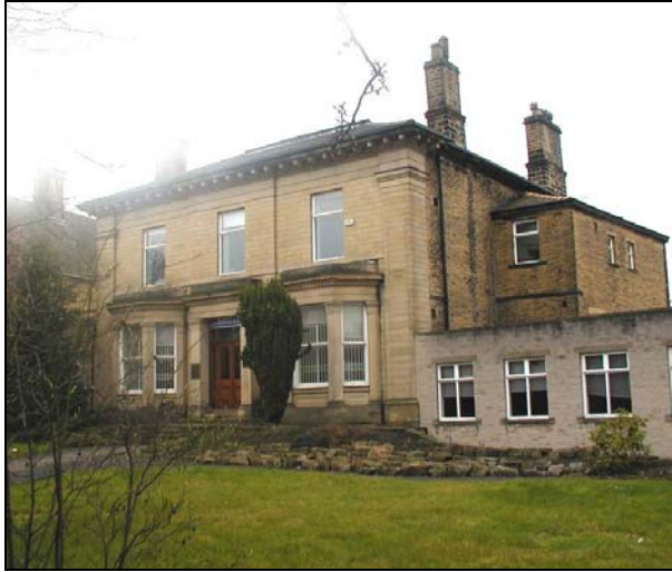
66 Little Horton Lane is an attractive Grade II listed Victorian villa. The unattractive extension to the right of the building is an incongruous addition.
