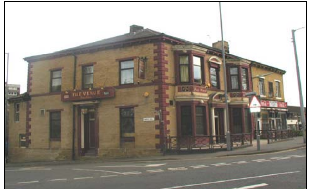
The Venue, located on the corner of Park Road and Little Horton Lane was formerly a villa but has since been converted into a public house.
