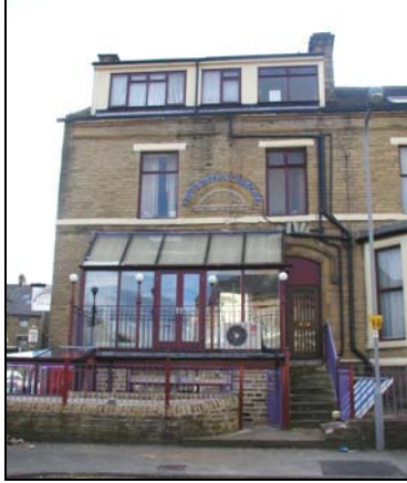
Many of the properties on Mannville Terrace have been converted from residential use into commercial use. The subsequent alterations have not always been sympathetic to the age and character of the building.
