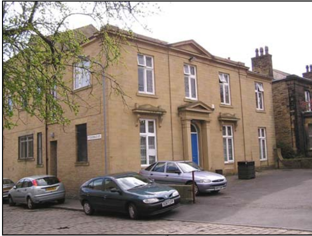
123 Little Horton Lane, a mid 19 th century listed villa has been built in a Greek Revival architectural style.
