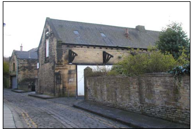
The stone building on Back Russell Street may have originally been a coach house but has recently been converted into office use.
