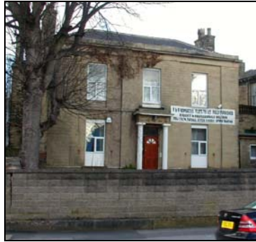
The insensitive replacement of the original sash windows to 115 Little Horton Lane, a Grade II listed villa, has undermined the historic character of the building.
