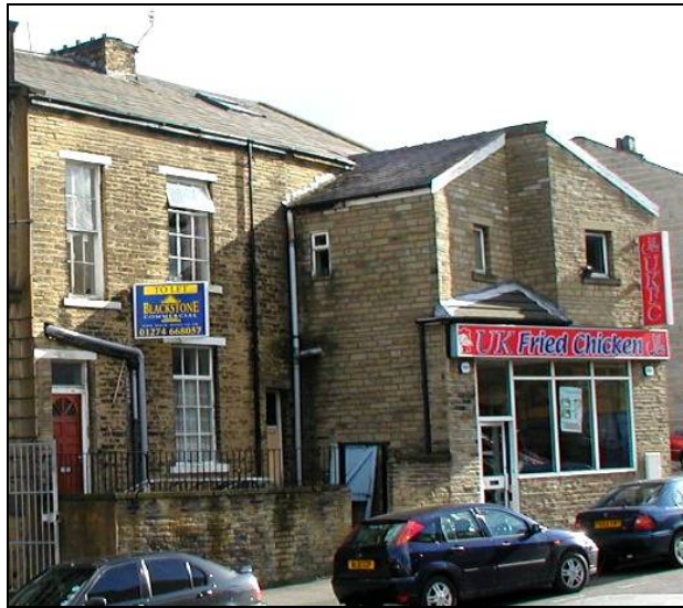
The modern rear shop extension to 8 Lansdowne Place is incongruous with the style of the pair of houses to which it is attached.
