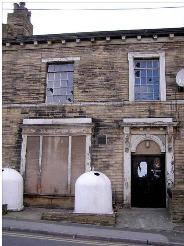
Part of the neglected and vacant 20 Lansdowne Place.
