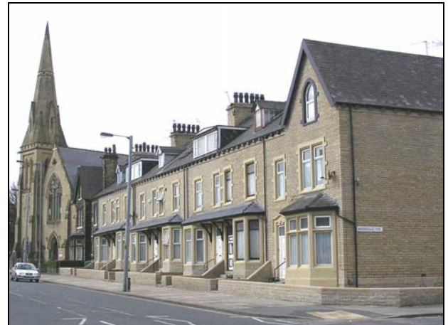
The vigorous stone cleaning of 82-96 Little Horton Lane has left the stone unnaturally bright.
