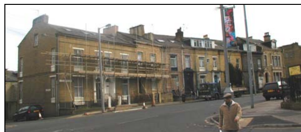
127-147a Little Horton Lane are aligned to the bend in the road and though have lost much of their original character, are of streetscape value to the conservation area.
