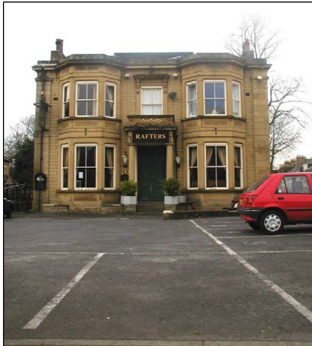
Large expanses of tarmac extending from the boundary right up to the building are detrimental to the setting of listed buildings and have a cumulative impact on the character of Little Horton.
