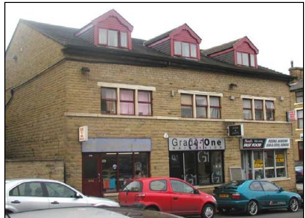
122a-122c is an inconsistently detailed modern building; the shopfronts are modern and poorly detailed whereas the first floor windows are a pastiche of the mullioned lights of weavers cottages from c.1800 - 1820. Neither detail is in keeping with the architecture of the Victorian suburb of Little Horton Lane.
