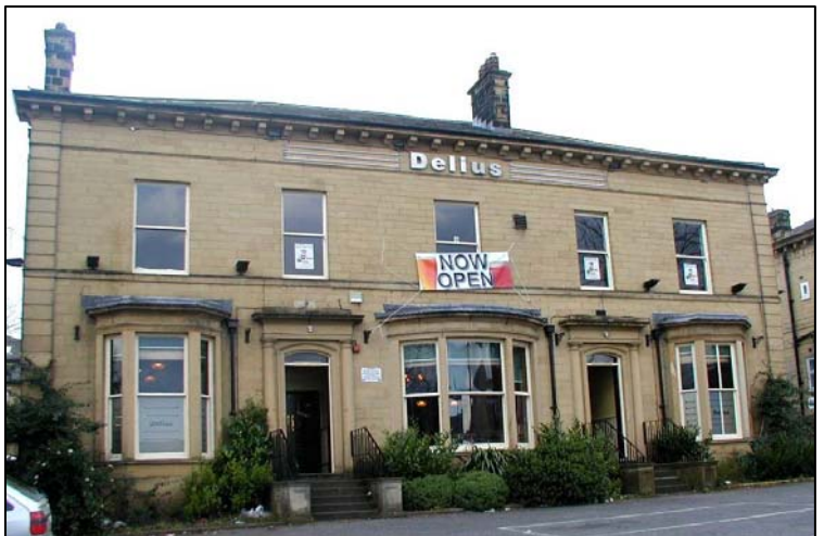
8-10 Claremont (Grade II Listed) is one of several pairs of villas along Claremont which share a five-bay frontage. This Classical style villa has recently been sensitively converted into a bar.
