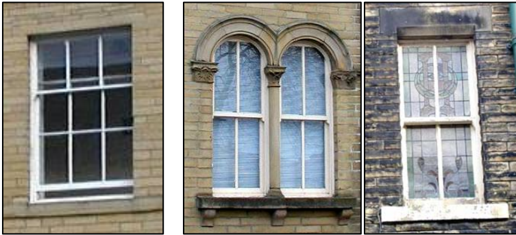
Various types of timber sash windows, which are important traditional details and should be conserved.
