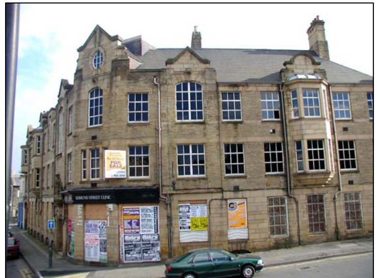
The former Edmund Street Clinic occupies a prominent position and this massive building is in an eclectic style.
