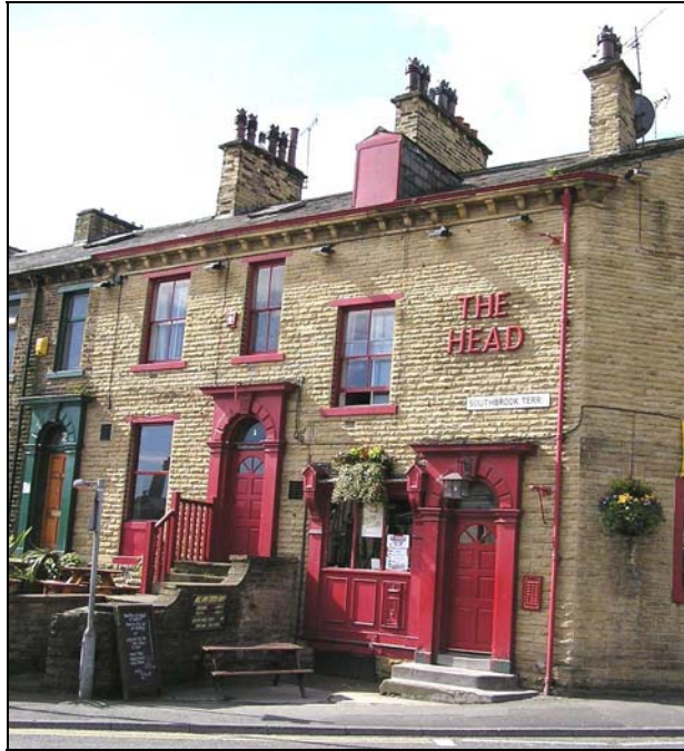
The Head is a well-detailed Grade II Listed public house at the end of Southbrook Terrace.
