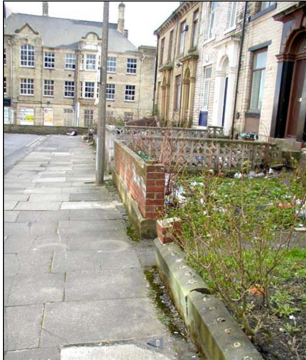
Poor pedestrian surfaces, unsympathetically altered boundary features and poor maintenance have a cumulative impact on the appearance of Grove Terrace and the surrounding streets.
