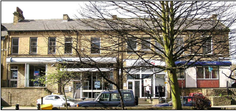
2-8 Mannville Terrace. Note how modern style shopfronts and signage have disfigured this row of four houses.
