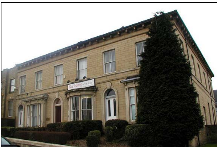
32-36 Little Horton Lane (Grade II Listed). These large houses have been converted to offices with minimal external alteration.
