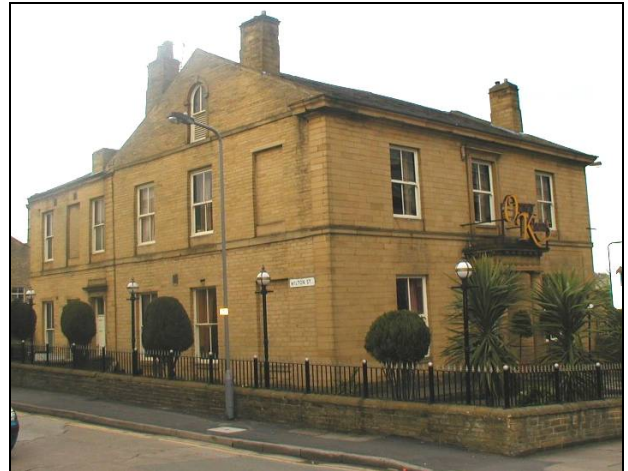
30 Little Horton Lane (Grade II Listed) was built as the home and surgery of a dentist. It has been sensitively converted into a restaurant.
