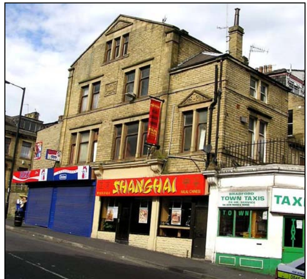
98-104a Morley Street are shops with unsympathetically modernised and secured frontages. The refaced elevation to 37 Grove Terrace (above the shops) incorporates pediment details and is dated 1915.
