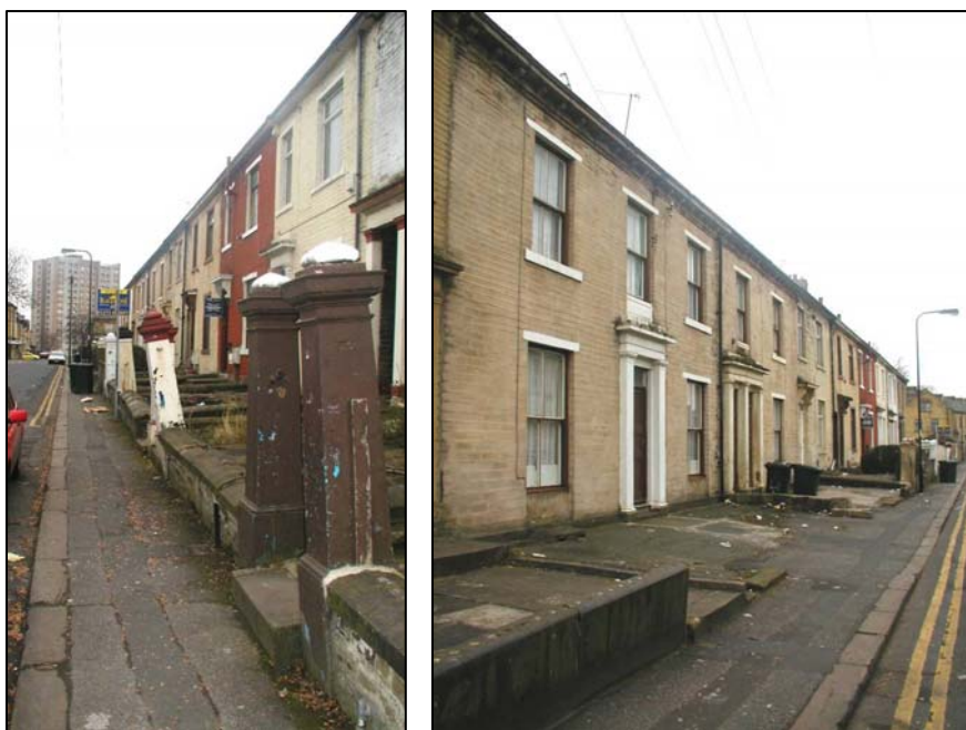
A number of coped stone walls with traditional stone gatepiers (all of which have been altered) line Sawrey Place (left), but in some instances, these details have been removed completely, much to the detriment of the appearance of the street (right)
