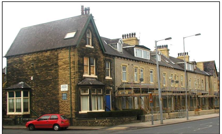
Stone cleaning not only disguises the true age of a building, but also creates unwanted contrasts between darkened and cleaned stone as shown here at Little Horton Lane.
