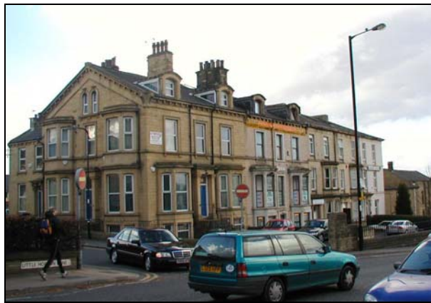
42-50 Little Horton Lane are prominent buildings fronting onto the main road.
