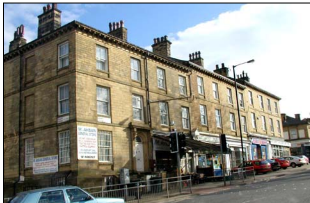
93-101a Little Horton Lane occupy a prominent position at the northern end of Little Horton Lane.
