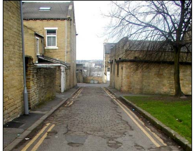
Above: The setted surface of Swan Street is reappearing as the tarmac surface becomes dislodged.
