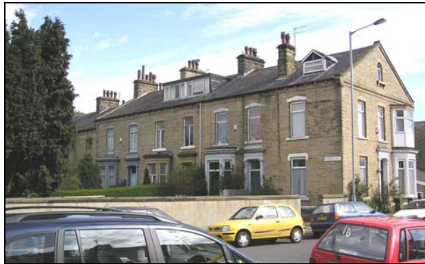
2-10 Russell Street are an attractive terrace of late 19 th century dwellings that are set back from Russell Street behind long, green gardens.
