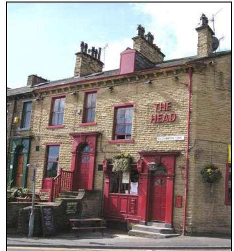
The Head public house, located on the corner of Southbrook Terrace, dates from the 19 th century and retains a number of interesting features.
