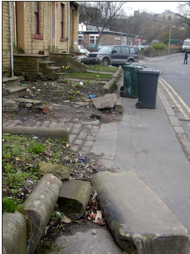
These collapsed boundaries at Claremont Terrace are in a poor condition and present a hazard to pedestrians. Note the stone kerb and setted way, two other surviving original details.
