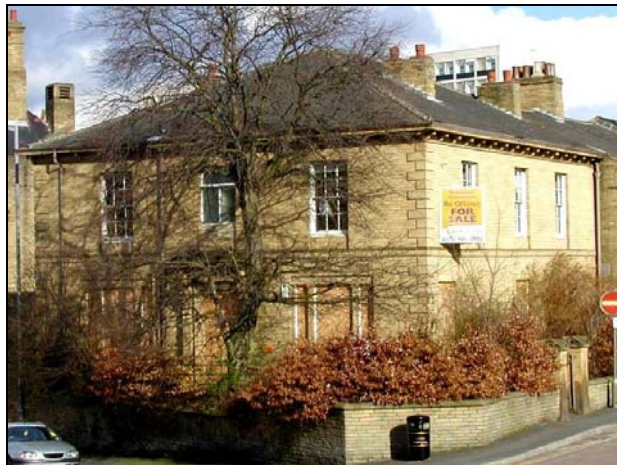
The vacant 30 Edmund Street (Grade II Listed) is a well detailed villa which is contemporary with the rest of the terrace that it is attached to.
