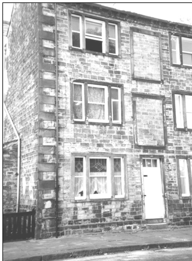
54 Little Horton Green is part of a block of Grade I Listed cottages built for cotton workers. The blocked loading doors over the doorway were originally used to move textiles in and out of the workshops on the upper floors.
