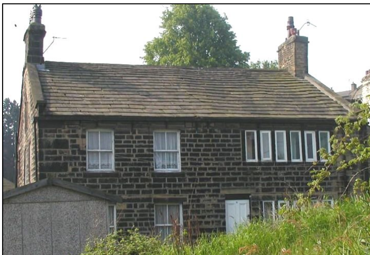
The right hand property displays the traditional rows of flat-faced mullioned casement windows found on houses and cottages built in the area in the late 18 th and early 19 th centuries. The left hand house was refenestrated in the late 19 th century with two-pane sash windows which are a typical detail of the time. The windows and four panelled door are important in upholding the historic appearance of the building.
