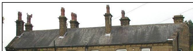
Below: Welsh slate roof and late 19 th century chimneys.
