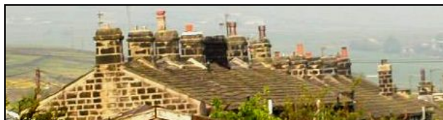
Above: Stone roof and early 19 th century chimney detail.
