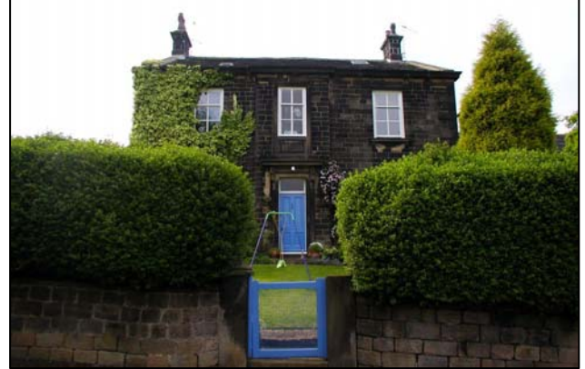
West Croft (key unlisted building)
