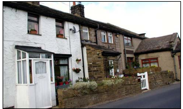
Alterations to the stonework such as the painted render, strap pointing and pebbledash render shown on these three houses undermines the group value and historic character of buildings. The changing of window and door detailing exacerbates the incongruous appearance of the group.
