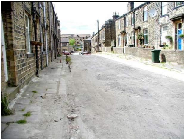
The unadopted Beatrice Street and the rest of the grid of terraces are historically unsurfaced and are in a poor condition. The York stone paving flags and kerbstones are also poorly maintained. Note how the long flat elevations of the houses and boundary wall give the street a consistent appearance and character.
