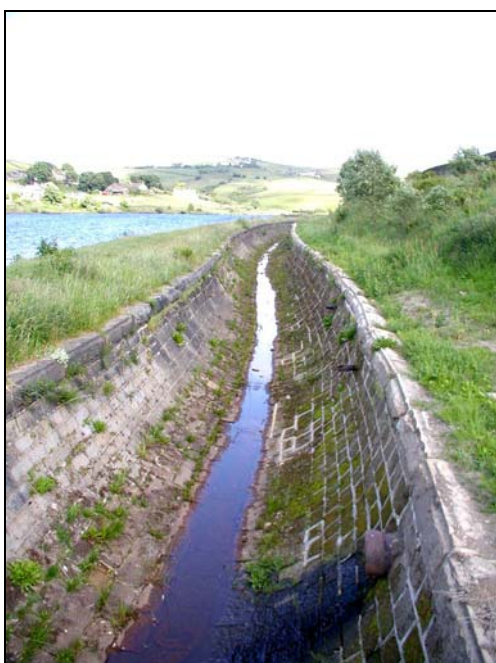
The weir feeds into a manmade overflow channel which is separated from the reservoir by a steep embankment which is topped by a footpath.
