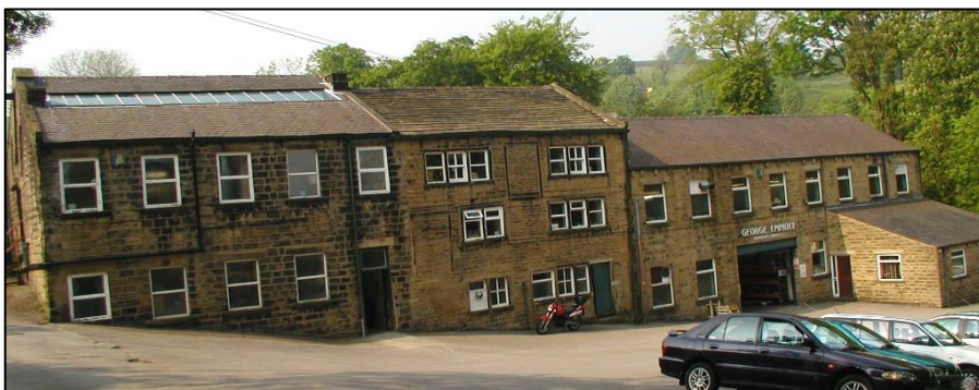
Wadsworth Mill (key unlisted building) is built in three distinct phases. The central section with blocked taking-in doors was built as a textile mill. In the mid-19 th century the firm switched to making springs and expanded the premises twice.
