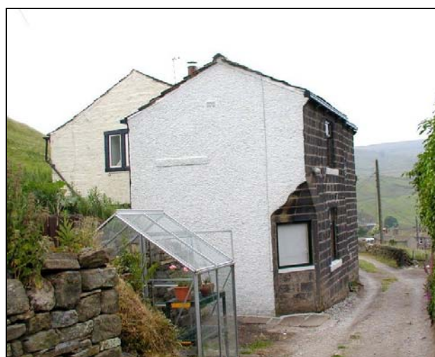
12 Bank (unlisted) has an unusual chamfered doorway (now partially blocked), suggesting that the building might once have been used for commercial purposes.
