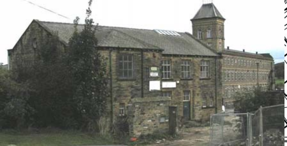
Apperdale Mill with Oaklea Mills in the background (key unlisted buildings).
