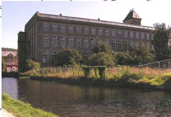
Oaklea Mills (key unlisted building).
