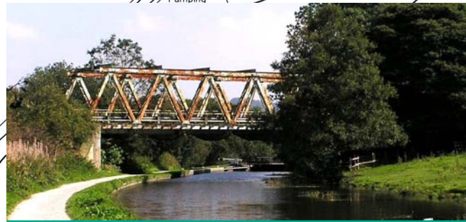
Western approach to the former railway bridge.
