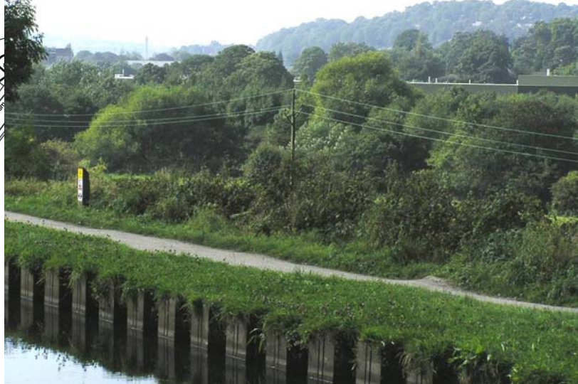
Metal piling along the canal bank near Buck Mill Lane.
