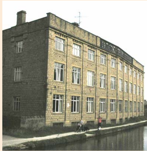
Dockfield Mills (key unlisted building), an impressive later mill of c.1900.
