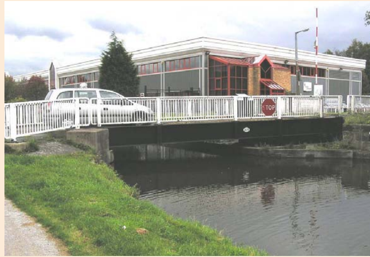
The modernised Oak Lane Bridge, with modern factory premises (outside the conservation area) in the background.
