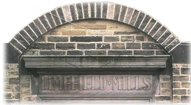
Far Right: Airedale Mills is a more or less complete canalside worsted mill. Contrasting with both the rural and suburban setting provided by the north and south sides of the canal respectively, the mills are an important industrial landmark with a direct association with the canal.
