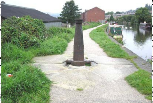
This iron upright is a remnant of a crane which stood on the former Wharf near Bank's Bridge.
