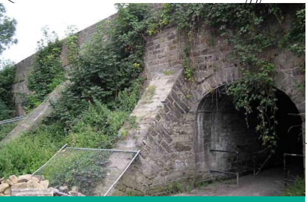
Silsden aqueduct (Grade II Listed) stands within Silsden conservation area.
