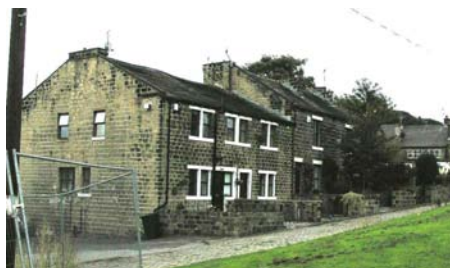
From the Top: It is proposed to alter the boundary of the conservation area around Esholt Sewage Works so that it follows a more legible line;
