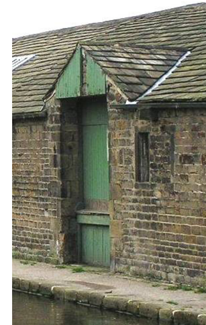
Above: Old warehouse, Stockbridge Wharf.
