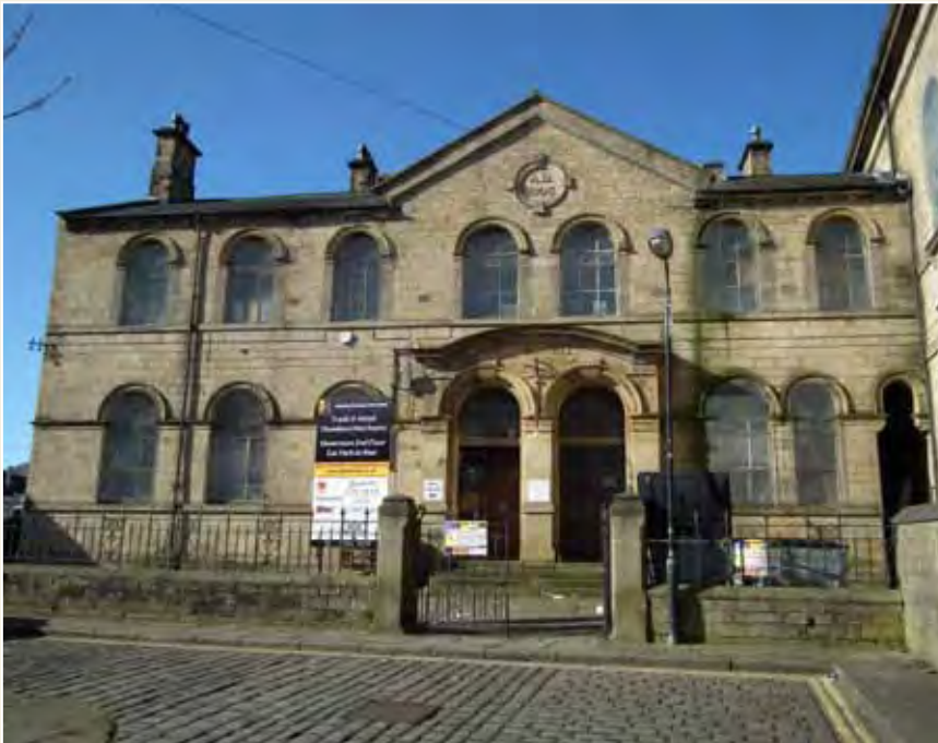
The former Sunday School on Temple Street, now a plumber's merchants
