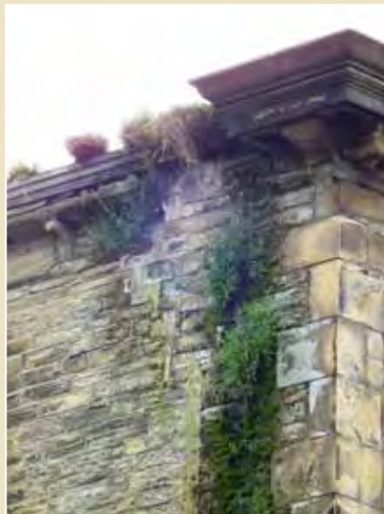
Damaged stonework and damp penetration caused by poor maintenance
