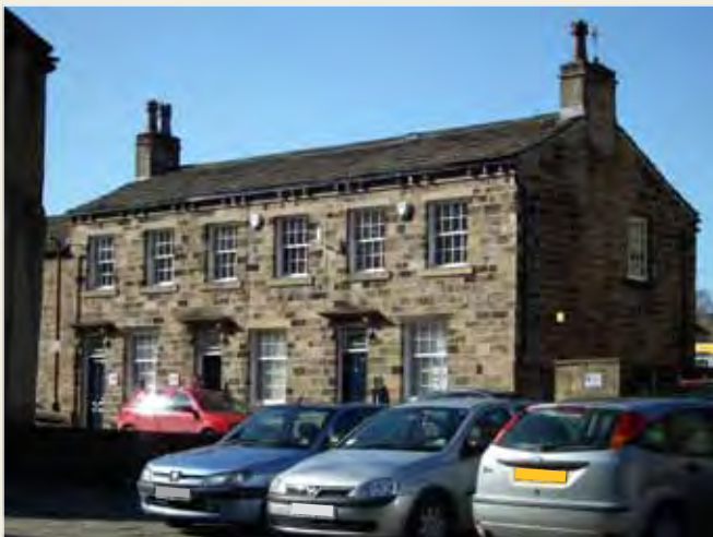
19-23 Temple Street (Grade II), with their characteristic 16 paned sash windows
