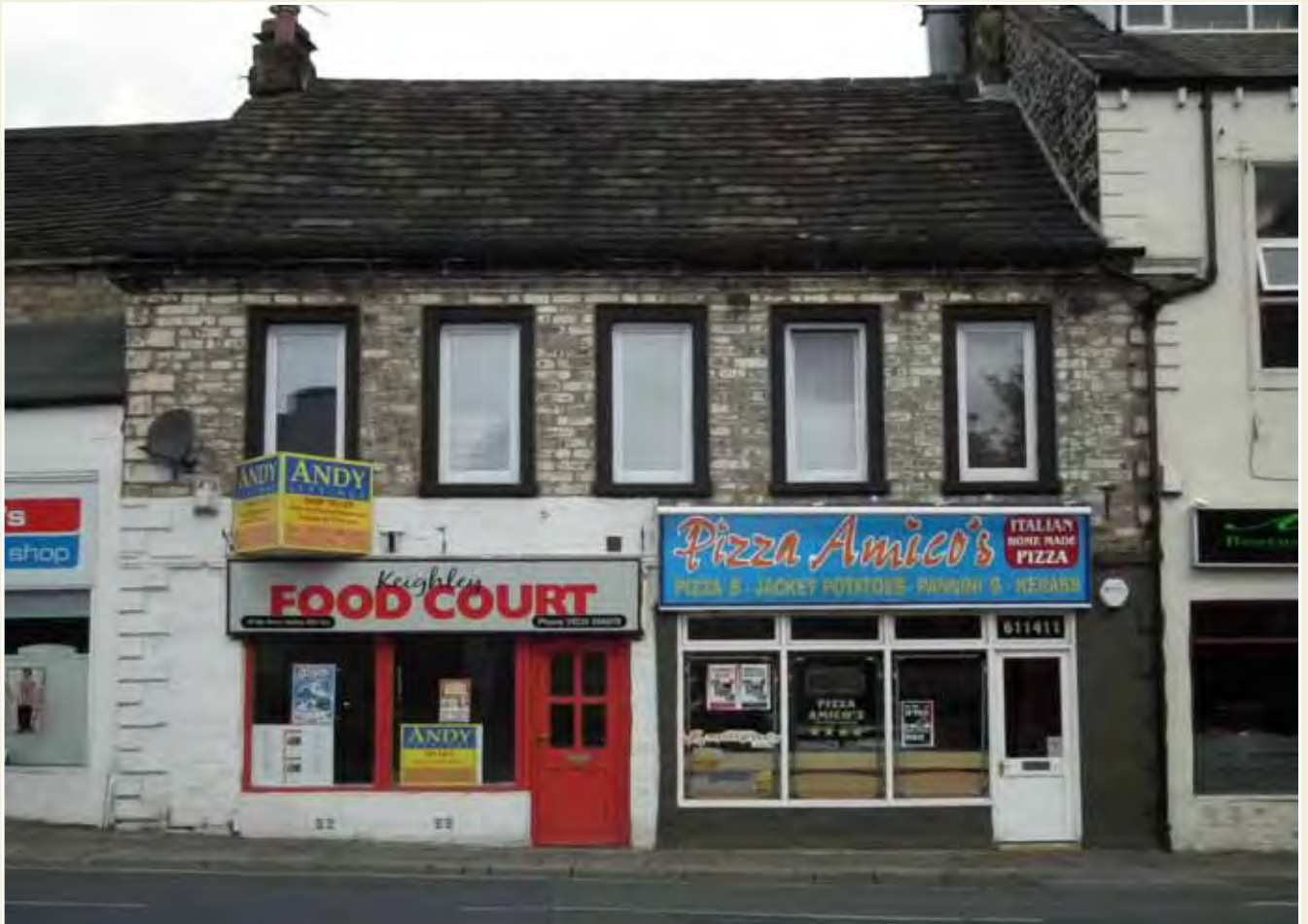
40-42 High Street (Grade II) is considered to be the oldest building in the conservation area, but sadly disfigured by the insertion of unsympathetic shopfronts, out of scale signage and upvc windows
