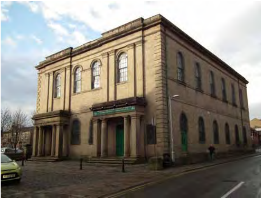
Mosque (Grade II) on Temple Street, a former Methodist Chapel
