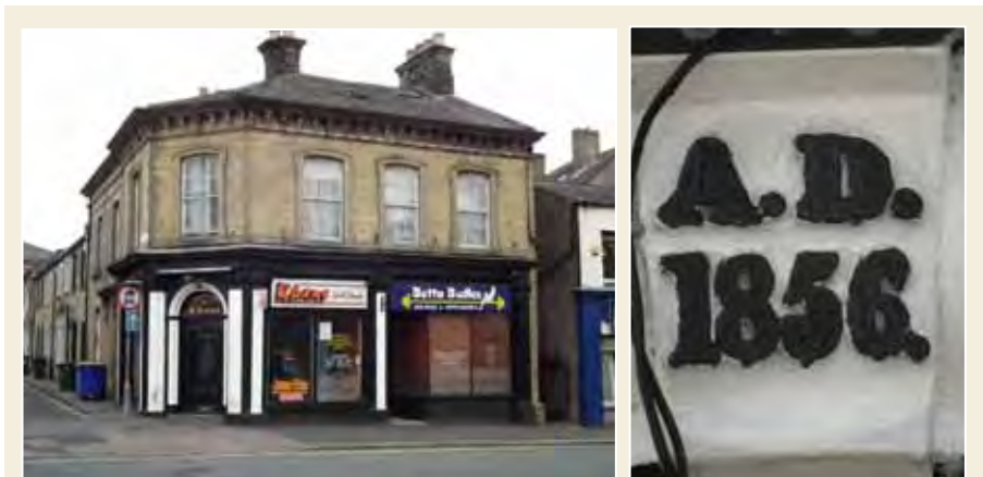
16-18 High Street, with a datestone of 1856 above the door
