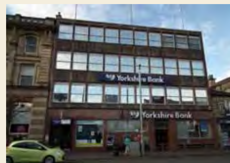
Later twentieth century buildings inserted into the terrace of stone buildings on North Street
