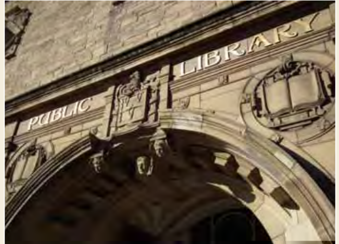
Keighley Library (Grade II) built with funding from Andrew Carnegie
