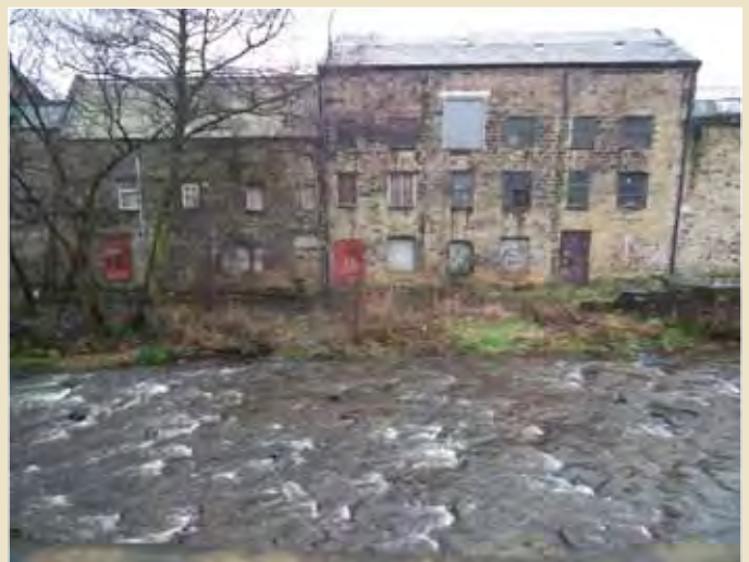
Buildings in poor condition on Beck Street
