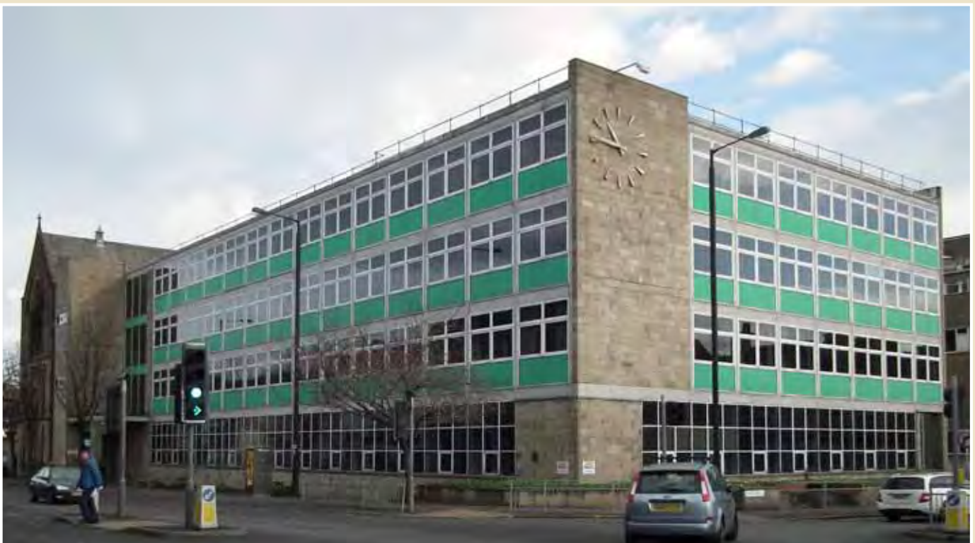
The former Keighley College building on North Street
