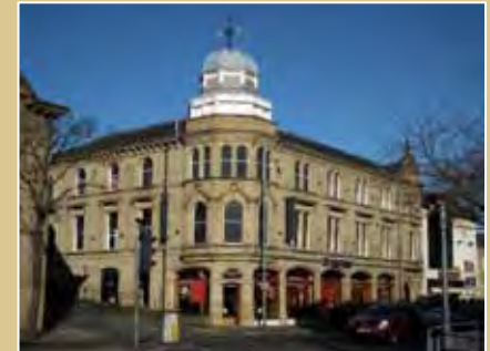
Top: 31 Church Street – the shop front has a large sash window
