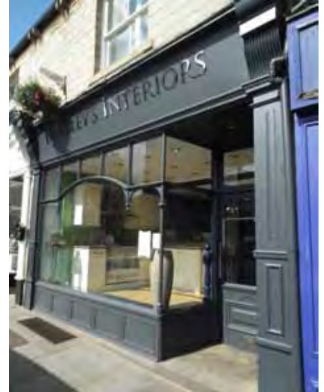
Well maintained traditional shopfront on Church Street with appropriate signage
