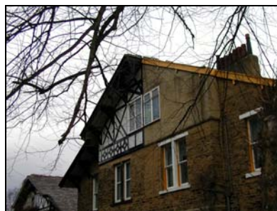
The loss of the timber detail and oversailing roof adversely affects the traditional appearance of the whole building which in turn is detrimental to the character of the conservation area.
