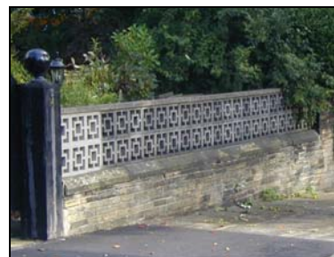
It is likely that cast iron railings originally stood on this stonewall. The use of concrete as a boundary treatment does not complement the character of the area.
