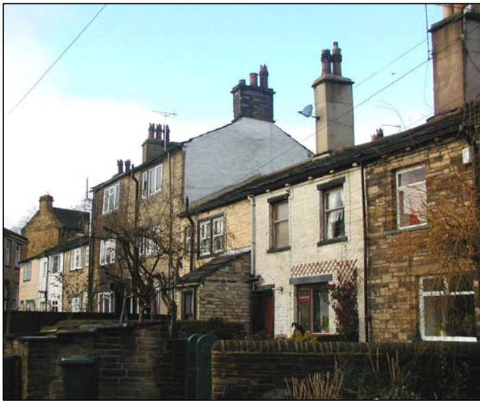
2-16 Liversedge Row. Numbers 6-16 are Grade II Listed, yet the painting of stonework, the removal of mullions and the replacement of traditional door and window details with modern style details have undermined the group and historic value of the row.
