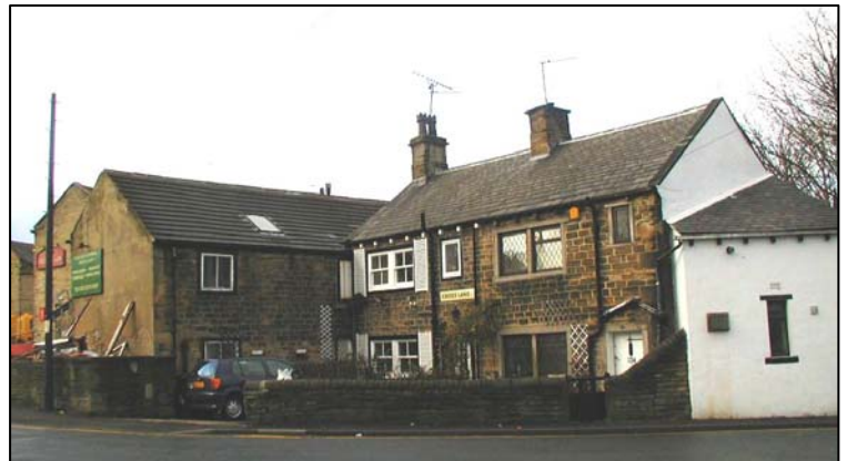
124-6 Cross Lane is a pair of cottages built c.1800. Note the rendered extension to 124 and the rear elevation of 6 Low Green which suggests that this building was once a row of cottages.
