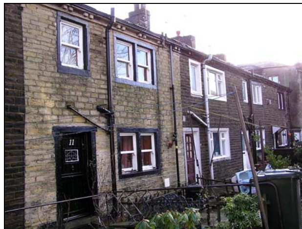
11-14 Cragg Lane is part of a Grade II Listed row of back-to-back cottages. Despite being listed, the appearance of the cottages has been altered and few original details remain.
