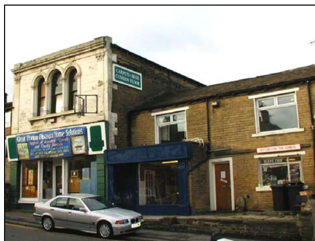
564-568 Great Horton Road were once the Number 10 Branch of the Great Horton Co-operative Society. The upper photo shows how the building appeared 95 years ago and as it did in 2003.
