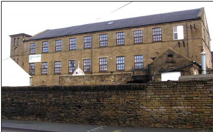
Jamilia Islamia Mosque was built in 1821 as Cross Lane Mill and is Grade II Listed.
