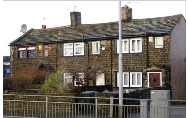
Above: 702-706 Great Horton Road are Grade II Listed, but their appearance has been altered through non-traditional windows and doors.
