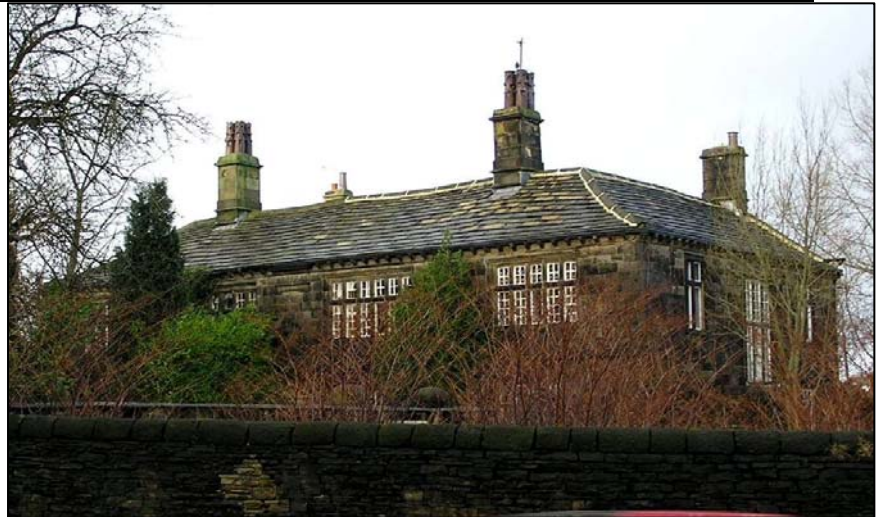
Most views of the Grade II* Listed 670-670a Great Horton Road are obscured by vegetation and the high garden wall which is Listed Grade II. Even so, the vernacular style transomed windows of the upper floors plus the stairlight on the eastern elevation are clearly visible. The appearance of the building has changed little since the drawing on page 12 was made.
