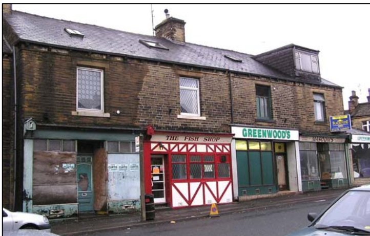
415-425 Southfield Lane. Note the contrast between the traditional shopfronts and the modernised ones.
