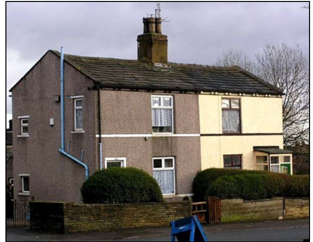
282-284 Southfield Lane have been extensively and unsympathetically modernised such that their appearance belies that these houses probably date from the late Georgian period.
