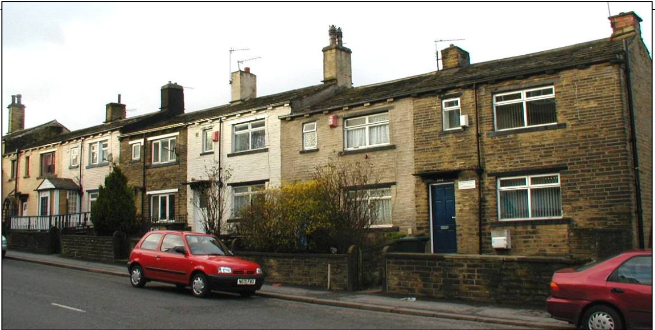
The painting of stonework, the removal of mullions, the different styles of unsympathetic glazing and other alterations have cumulatively undermined the group value and historic character of this row of cottages.
