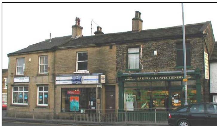
499-503 Great Horton Road. The traditional style re-fitted shopfront at 503 contrasts with the modernised shopfronts at 499-501.
