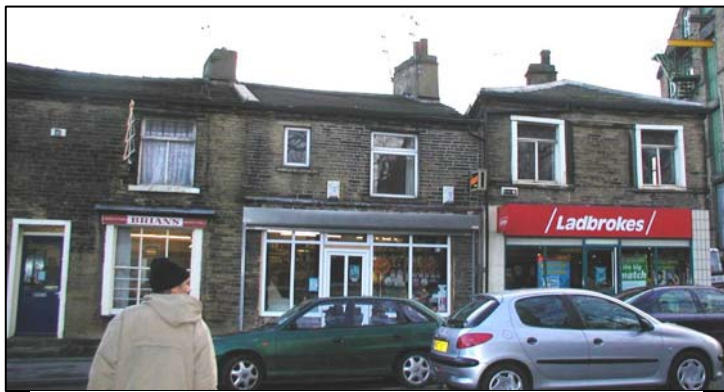
515-519 Great Horton Road. Note how the traditional shopfront details of 515 are contrasted in terms of scale, layout and materials to the modern shopfronts of 517-519.
