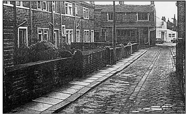
Cragg Lane as it appeared in 1974. The overwhelming majority of the traditional street surfaces have been removed, while the uniformity of the boundary walls has been undermined through partial demolition and alterations.
