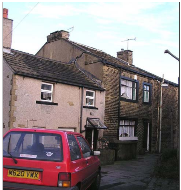
Below: 10-12 Dracup Road is also Grade II Listed, but here the rendering of stonework and the removal of mullions undermine the historic appearance of the group
