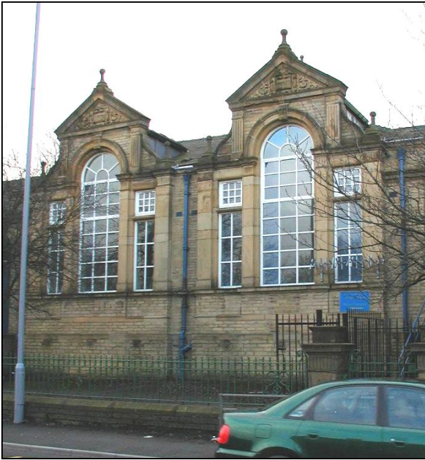
The pair of gable-fronted bays on the northern block of St Oswald's CE Primary School shows the mixture of Classic and Queen Anne Revival architecture of this Grade II Listed Building.
