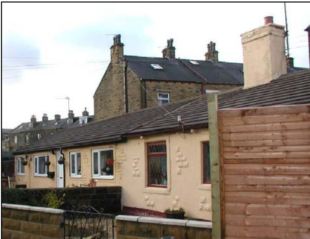
2-4 Bartle Square have been modernised such that they have no traditional details.
