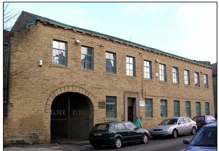
This warehouse on Bartle Lane is all that remains of the Grade II Listed Lane Close Mills
