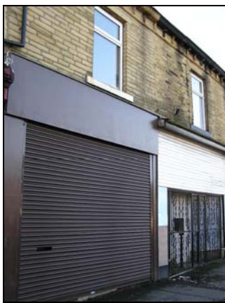
Shops should be made secure in a way that is appropriate and sympathetic to the historic buildings the shops occupy to create a more traditional and coherent street scene along the main shopping parades.
