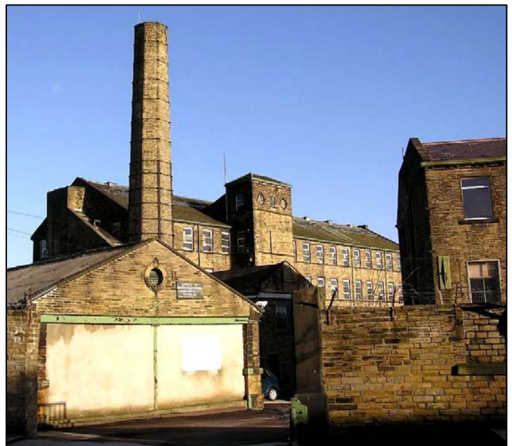
The large mass of the main shed at Harris Court Mill is complemented by the range of stone outbuildings and ancillary sheds at the complex. Their group value and impact on the character of the conservation area means that they are key unlisted buildings.
