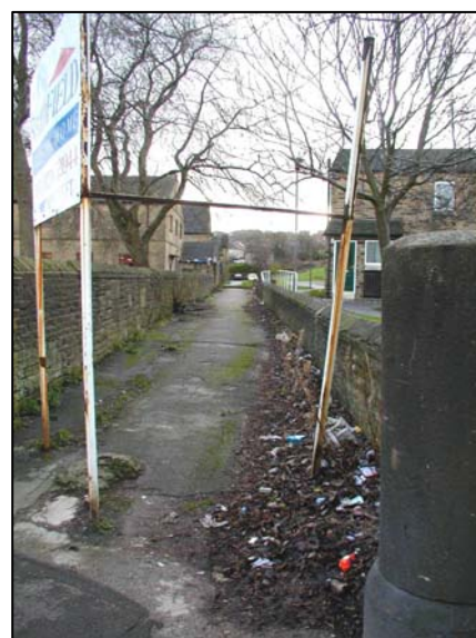
The footpath leading to Southfield Nursing Home is marred by the large sign at its entrance, litter and collapsed sections of wall.
