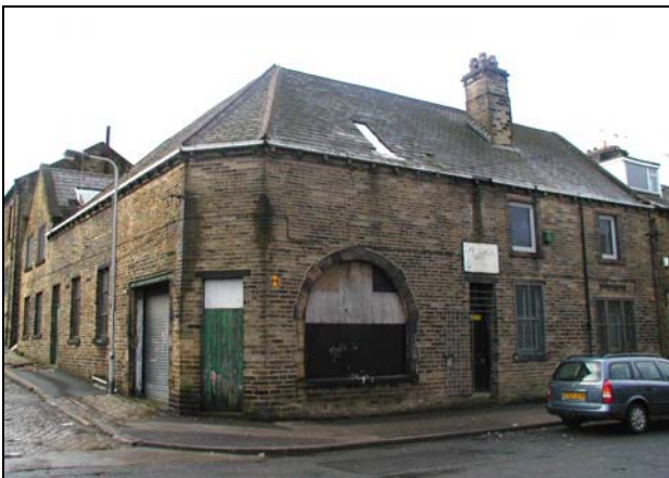
18-20 Low Green Terrace (key unlisted building). There was originally a quoined round-headed shop window either side of the corner doorway and the windows were a mixture of sash windows and fixed industrial windows.
