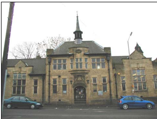
Great Horton Library is a unique Edwardian style civic building and is a key unlisted building of the conservation area.
