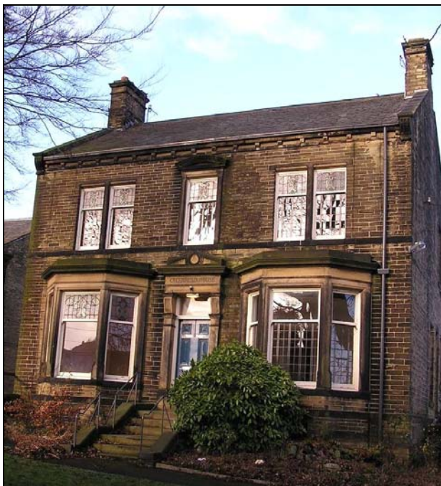
Greenfield House is a key unlisted building. The symmetrical villa retains original door and window details.
