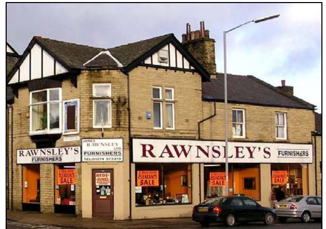
The appearance of 632 Great Horton Road has been altered through the modern shop windows inserted at ground floor and the out of proportion modern signs.
