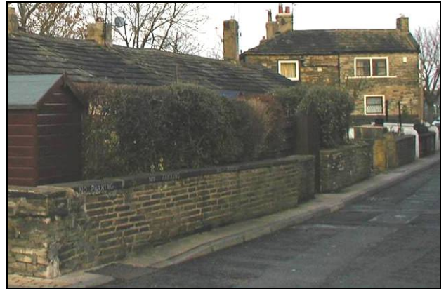
Traditional, coped stone boundary walls strengthen the traditional character of streets and folds.
