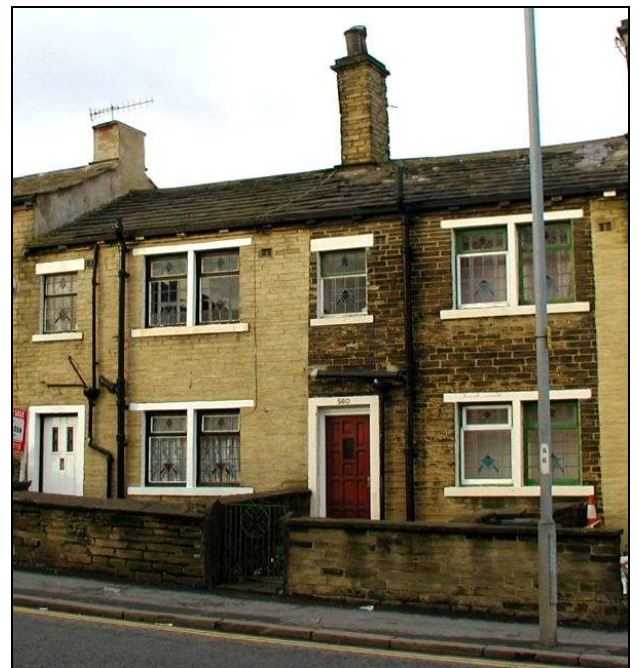
If it were not for the cleaning of stone and replacement of doors, these two cottages would look identical. The paintwork to the openings also stands out quite strongly.
