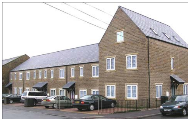
Poorly detailed, bland modern housing at Kingswood Street
