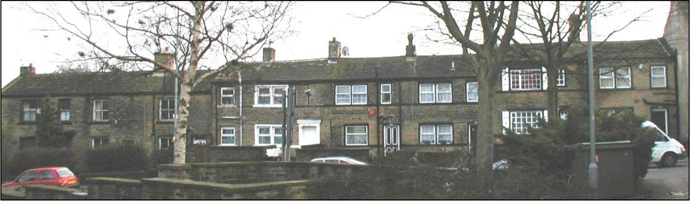
The unity of the stepped cottages at 437-449 Great Horton Road (Grade II Listed) is reduced by the replacement of most of the traditional door and window details with modern ones and the painting of stonework. The larger and later 437 is on the far left and with its cottage at 439 retains traditional sash windows.
