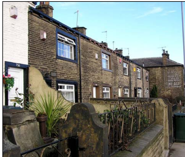
740-750 Great Horton Road is part of a longer gently stepped row of early 19 th century cottages. All cottages lack original details and some have been cleaned or painted.
