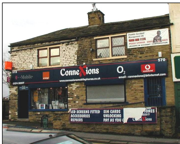
570-572 Great Horton Road. The shopfronts and signage of this building are completely inappropriate.
