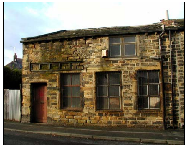
78 Cross Lane (key unlisted building). This unusual vernacular building is apparently still used as a foundry.
