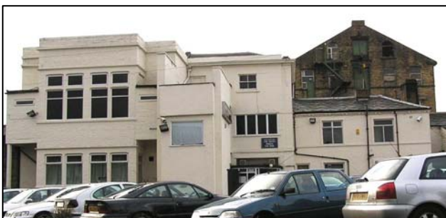
Great Horton Working Men's Club has been altered drastically during its lifetime such that little of the original mill master's dwelling (shown above) remains.
