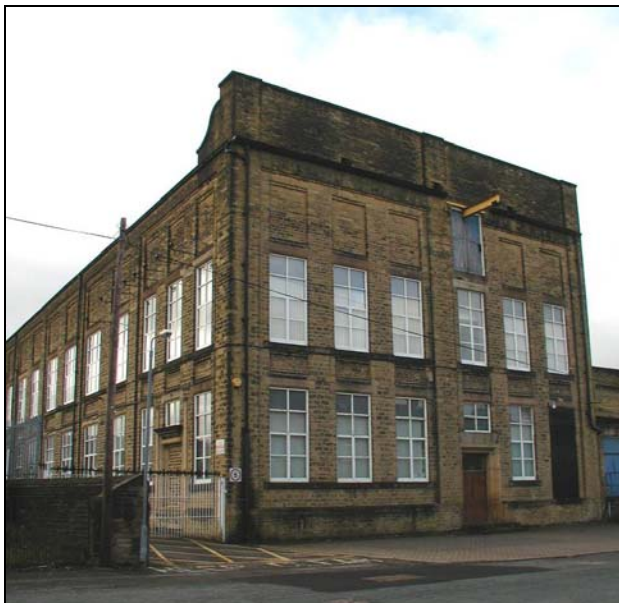
Westcroft Mill is one of a handful of mill complexes close to the conservation area. The sight of massive stone buildings such as this shed reinforce the character of the conservation area.
