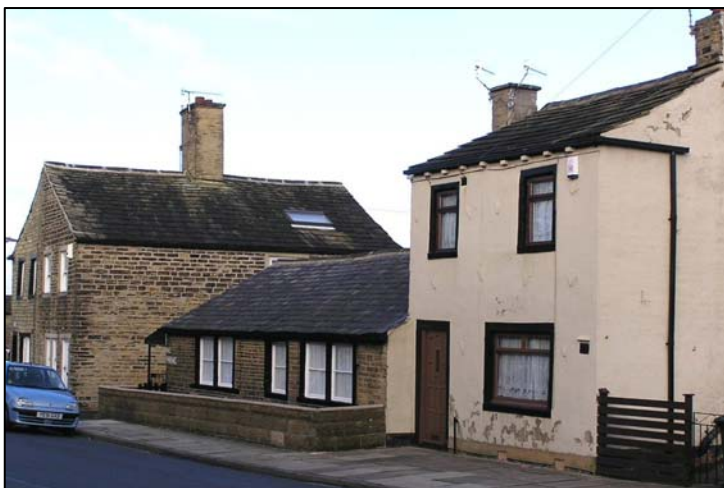
14-22 Dracup Road (Grade II Listed) is a disparate group of early 19 th century cottages made more disparate by unsympathetic alterations to some of the properties.
