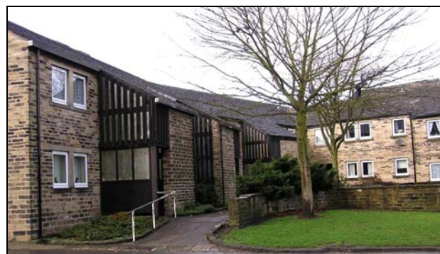
Hunt Yard. Although the catslide roofs and the use of traditional stone and timber are good details, the poor and plain detailing and materials elsewhere reduce Hunt Yard's contribution to the conservation area.
