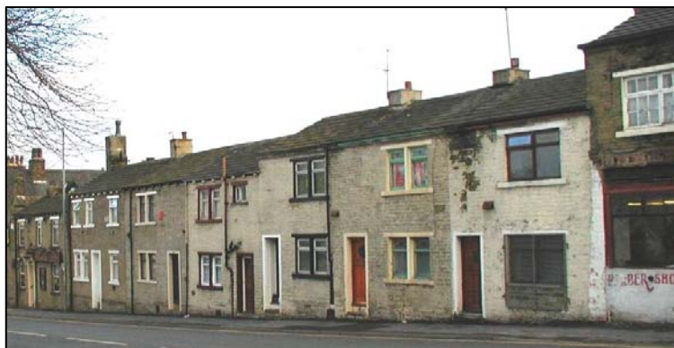
397-413 Great Horton Road are early 19 th century cottages which lack their traditional character due to the painting of stonework, alterations to chimneys and modern door and window details.
