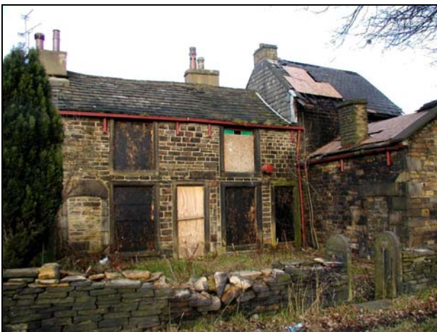
Dated 1657, but with early 19 th century alterations, the Grade II Listed 7-9 Cousen Place is presently empty and in a poor state
