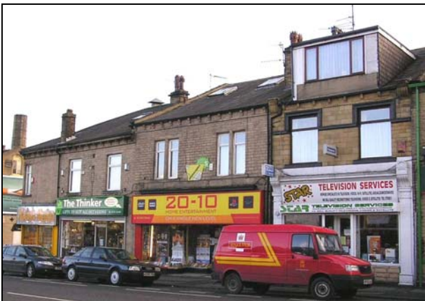
555-563 Great Horton Road is a parade of shops which is let down by incongruous shopfront modernisations and a dormer window which give the row a very disjointed appearance.
