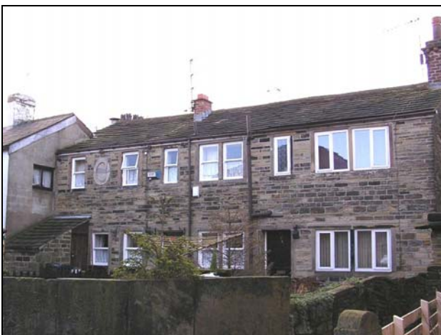
724-728 Great Horton Road. Three early industrial cottages dated 1732 and Listed Grade II with the other cottages around the fold.
