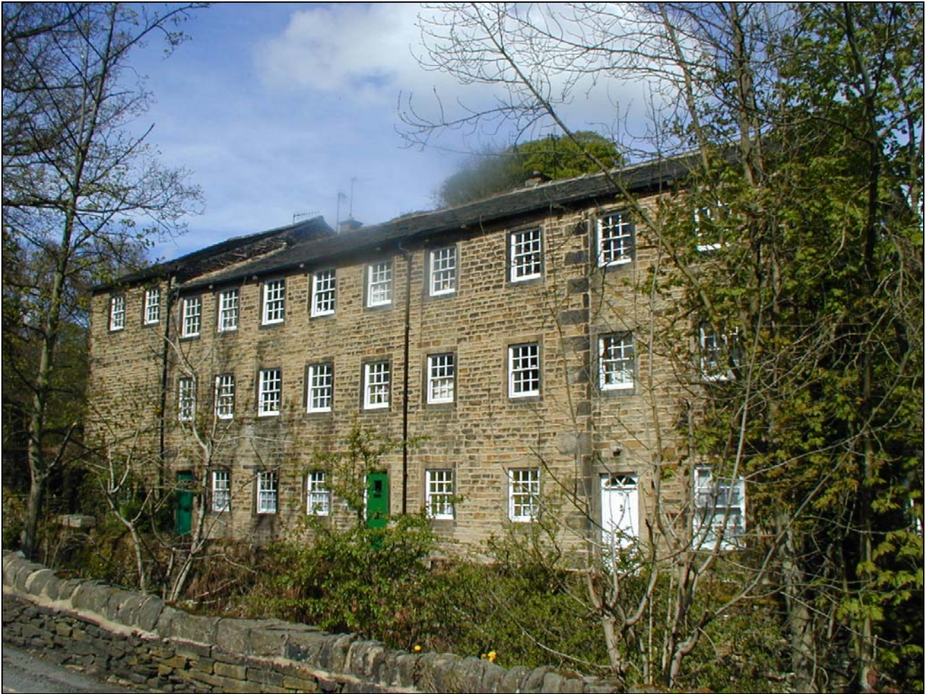
The Grade II Listed former Rag Mill is now three dwellings, but retains much of its traditional, industrial appearance. The mill chimney was unfortunately demolished in 1971 when the mill was vacant.
