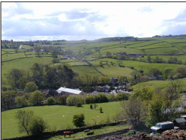
This view of Goose Eye from Laycock shows the importance of the fields which provide the setting of the conservation area. The mature trees which envelope Goose Eye are of high value to the conservation area.
