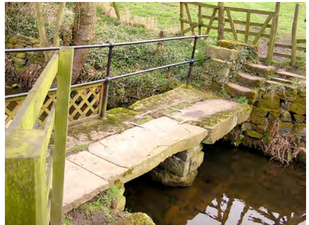
This clapper bridge over Eldwick Beck shows that this route is of some antiquity. The bridge helps to give the area a rural feel.
