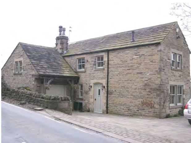
Huntsman's Cottage has been significantly remodelled and extended, but the quality of the design, materials and build has made the additions organic rather than intrusive.
