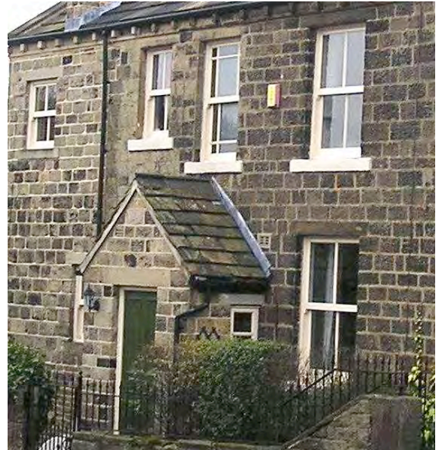
Timber sash windows and a four panel timber door at 136 Otley Road. These details make a particularly strong contribution to an otherwise quite plain façade.
