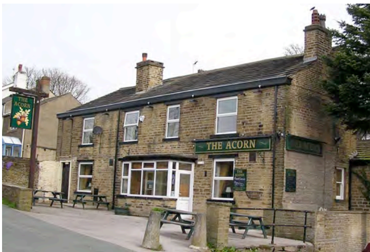
An inn dating from c.1820, The Acorn retains much of its character, but alterations such as uPVC windows and porch have undermined its traditional character.
