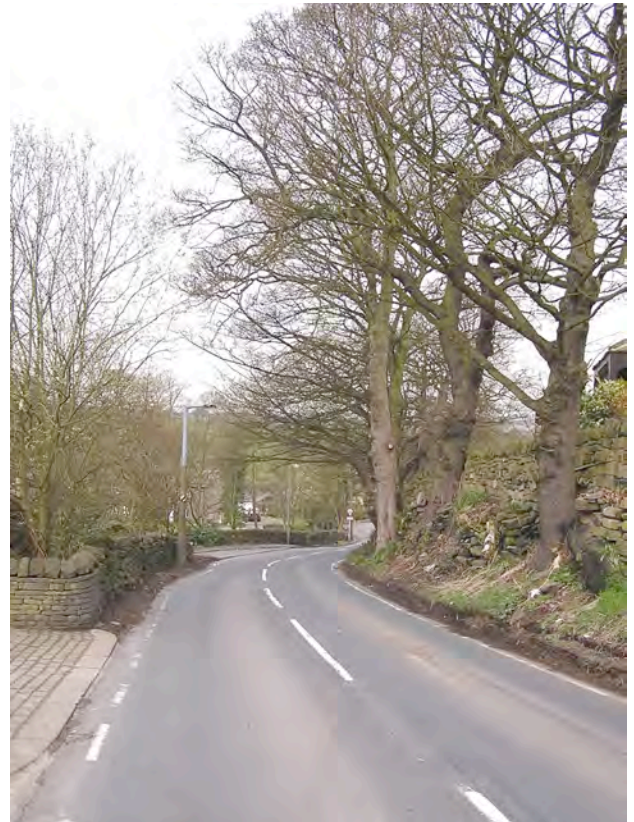
Spring Lane has an irregular width and course. In places it is bounded by verges like the one on the right, which contains mature trees. These different ingredients create a characterful street scene.
