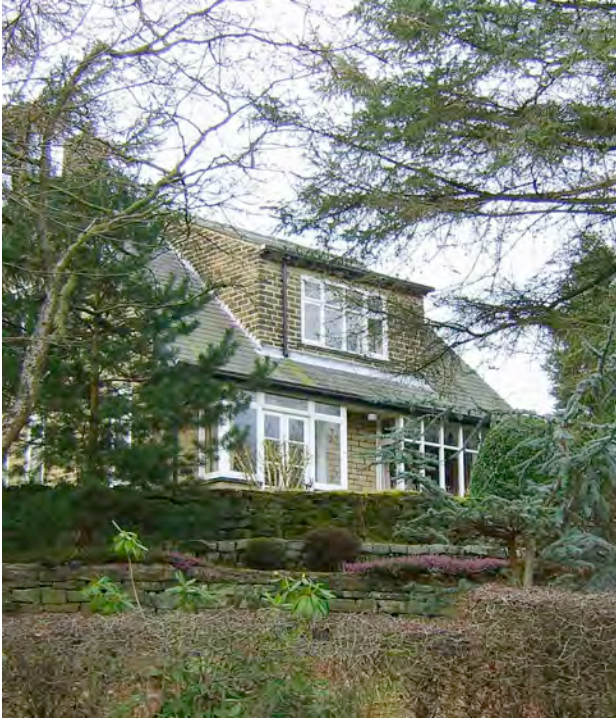
Glenside House (key unlisted building), may be a 1930s house, but it is a far from typical one owing to its unusual large central dormer set into the steeply pitched roof.
