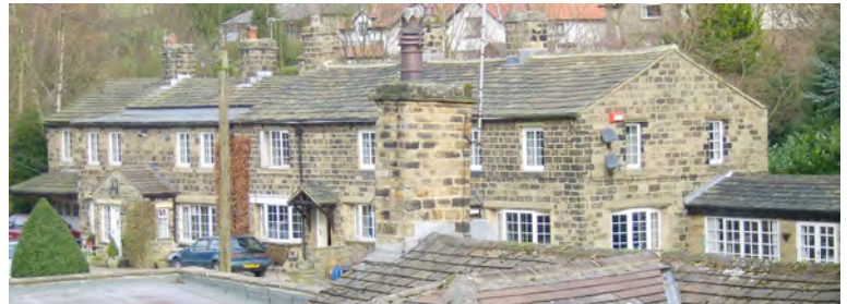
10-18 Eldwick Beck, although altered and now two dwellings, were built as a terrace of workers' cottages associated with Eldwick Beck Mill and they still from a distance look like a terrace due to the regular rhythm of chimneys and openings.
