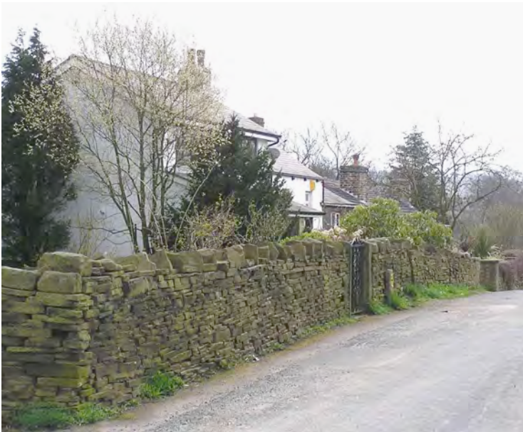
These traditional dry stone walls give a visually pleasing and consistent boundary to The Green. The dry stone detail harks back to the use of the land as a field before these houses were built.
