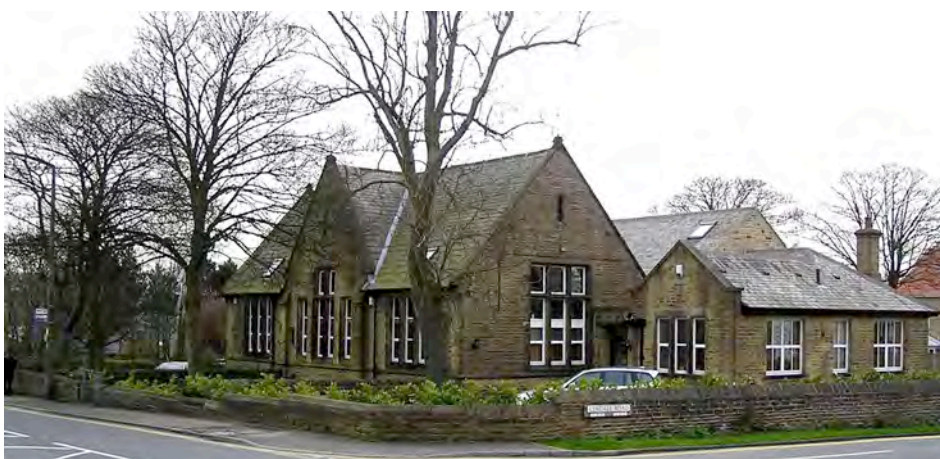
The Old School on Otley Road (key unlisted building) was built in c.1877 and served Eldwick Beck, High Eldwick and suburban Eldwick. It has been sensitively converted into three dwellings.
