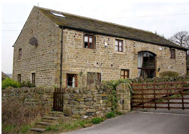
18 to 20 Paddock Lane (key unlisted building). Probably dating from the late 18 th or early 19 th century, this was originally the barn to Spring Farm and is now two dwellings.
