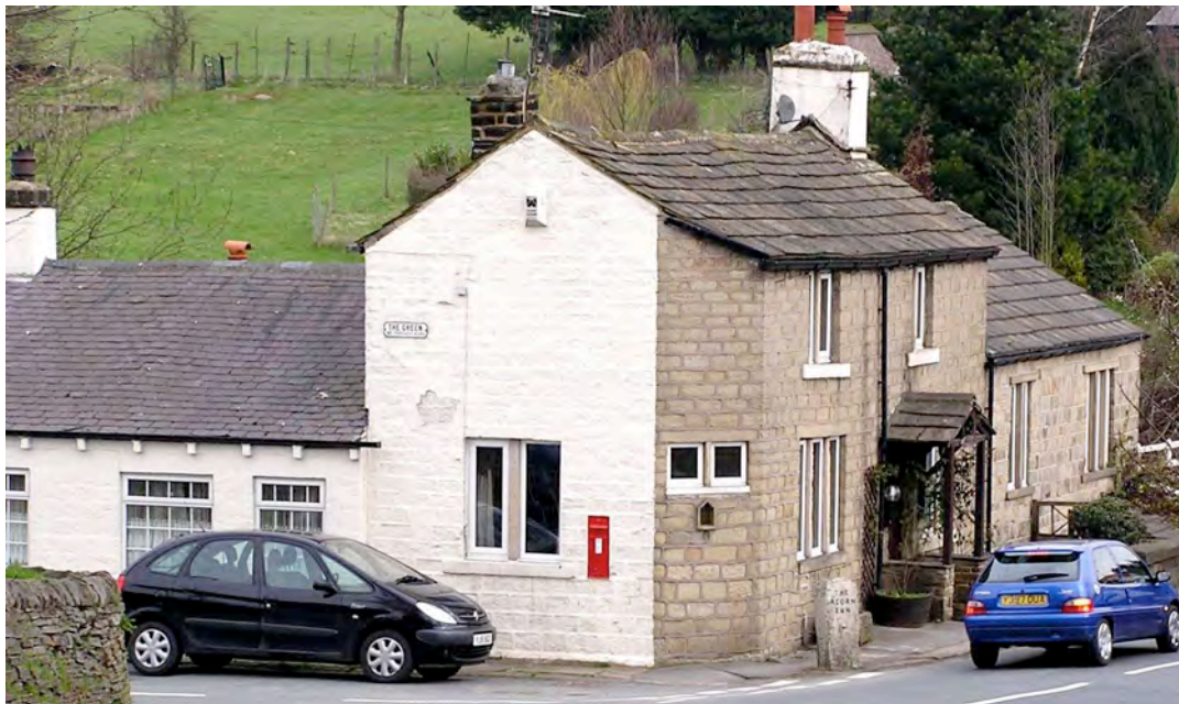
Bridge Cottage and 1 The Green. While chimneys and traditional roofing materials remain in situ, the painting of stonework, an inappropriate pointing detail and modern windows detract from an attractive, picturesque corner.
