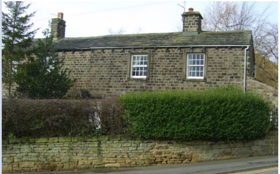
Main Street - traditional features retained such as stone slate roof and timber sash windows.
