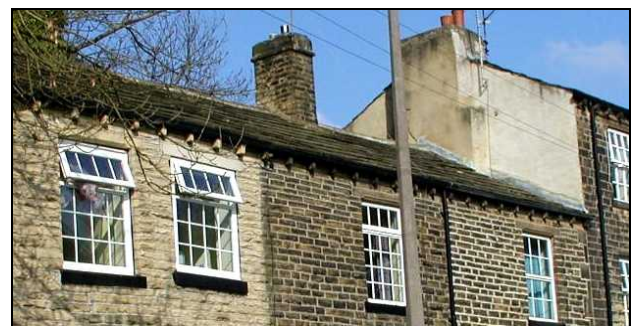
The stone wall of the middle property is as it should be, while the property on the left has been stone cleaned while the property on the right has a surfeit of mortar, giving this row an inconsistent appearance. The rendered gable to the right is uncharacteristic of the conservation area as stone elevations are traditionally bare.
