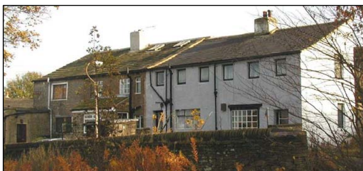
2-6 Tenter Hill (unlisted) have undergone extensive unsympathetic alteration, including the rendering and painting of stonework, the insertion of modern door and window details and the replacement of stone roof slates with modern tiles.
