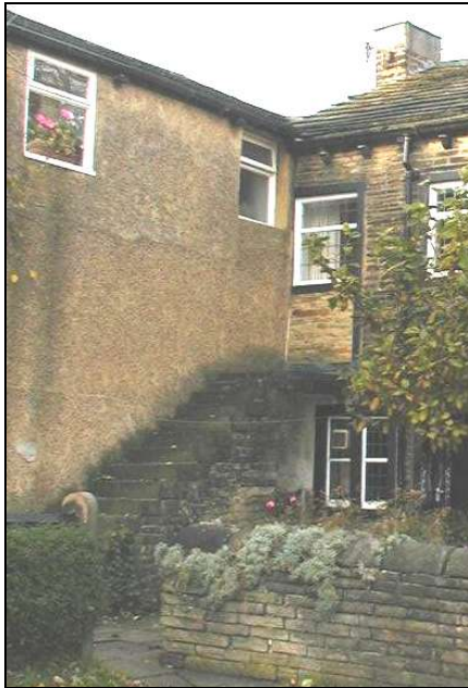
Built as the residence of a Maltster in c.1780, Maltkiln House retains an external stone staircase which formerly led to a workshop or storage room. Note the unsympathetic modern windows and rendered chimney to this Grade II Listed building and the rendered back wall of the cottages at Town End Road.
