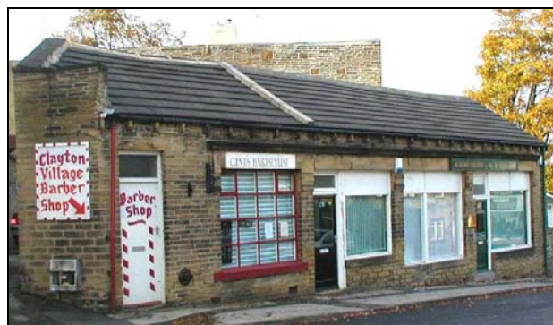
2a and 2b Clayton Lane (unlisted) retain traditional stone shop front details such as a long corniced fascia supported by consoles.
