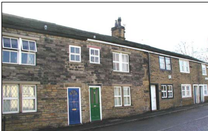
237-245 Bradford Road (Grade II Listed). The join between the original 18 th century house and the later cottages is indicated by the quoins to the left of the drainpipe.
