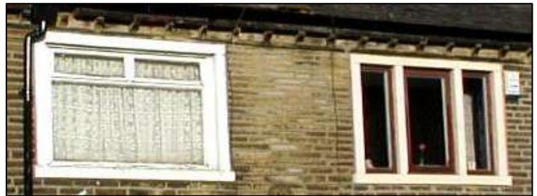
Replacement windows should respect the original or traditional appearance of the building. Both of these replacement windows lack the traditional detailing, while the insertion of that on the left has occasioned the removal of the mullions.
