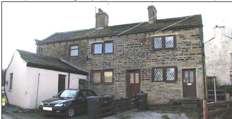
12-14 Back Fold and 2 Town End Road (left) are an early 19 th century rebuild of a mid-18 th century building and have a mixture of details from these dates, plus unsympathetic modern interventions such as the rendered single storey element of 2 Town End Road and the modern style windows.
