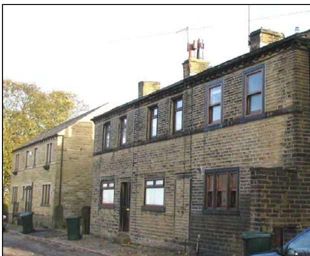
6-12 Broadfolds. Note the impact that the unsympathetic modern windows at number 8 makes on the elevation of the Grade II Listed 6-10 Broadfolds. The modern 12 Broadfolds mimics the fenestration and architecture of a traditional pair of cottages.
