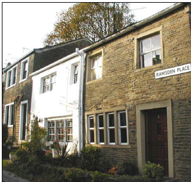
The painting of elevations and the margins of openings can seriously undermine the coherence of a group of buildings.
