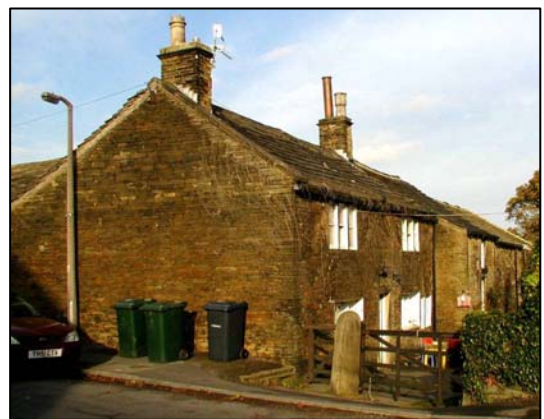
Town Bottom Farm (Grade II Listed) has a timber frame which dates from the 16 th century which was later encased in stone. To the right and projecting forward is a 19 th century element which links the farmhouse to a barn.
