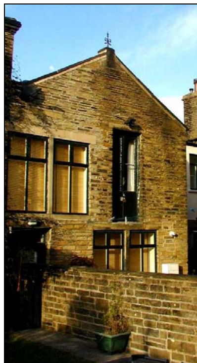
The Workshop retains much of its original pre-conversion character, particularly as the old timber loading door has been retained and glass panes inserted. The iron finial is an unusual decoration.
