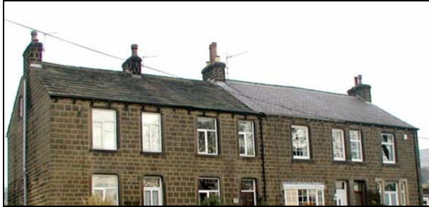
Stone slates and blue slate are both natural roofing materials and complement the stone of buildings in the conservation area.
