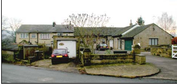
The rear elevations of Ivy Bank House, Cottage and Wynyates faces northwards towards the lane.
