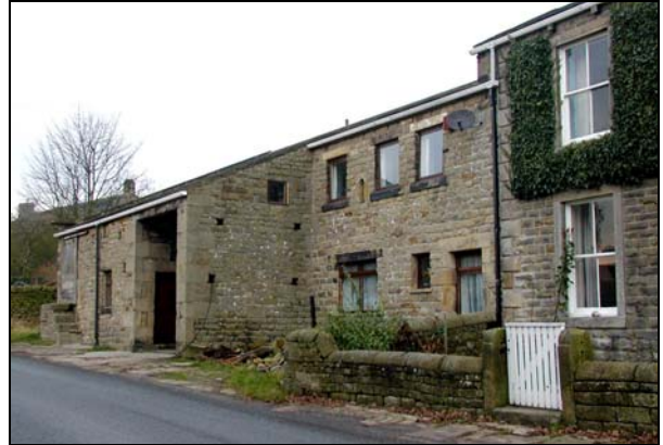
Croftend (key unlisted building) comprises of a small cottage adjoining a barn. Both are stone built and share a single stone slate roof.
