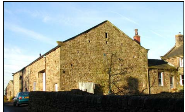
The western gable end of the barn lacks any openings other than the small breather holes that allow air to circulate.
