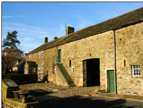
Sycamore Farm and barn (Grade II) listed. Photograph taken from listed building archives.
