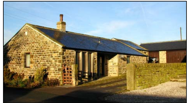
The single storey barn to the west of Ashwell Farm is now in residential use.
