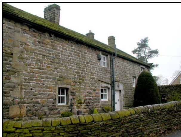
Rear elevation of Sycamore Farm and barn. Photograph taken from listed building archives.
