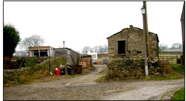
The site on which the caravan is located would benefit from a tidy up. Planning permission has recently been granted for the construction of a new dwelling in place of the ruined cottages.
