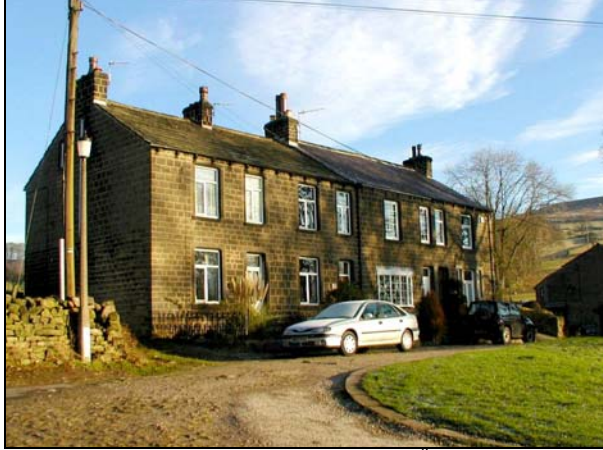
The Terrace is a row of four early 20 th century houses that are partly roofed in stone and partly in blue slate.
