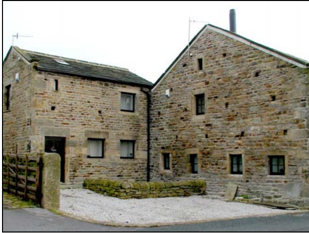
The stable, set back behind the gable end of the barn forms part of the Grade II listed group of buildings at Ashwell Farm.
