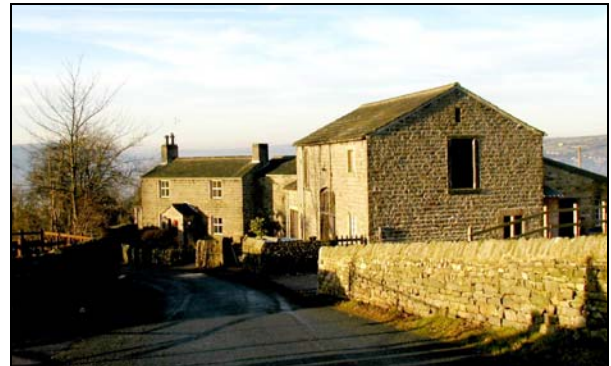
High Brunthwaite, to the east of the conservation area is an attractive hamlet located high up on the valley slopes.
